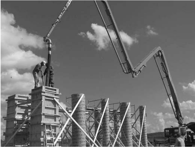
Figure 38. Column casting.
