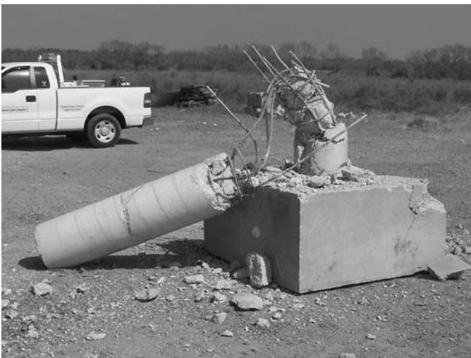
Figure 63. Local damage Test 3: Column 1A1.
