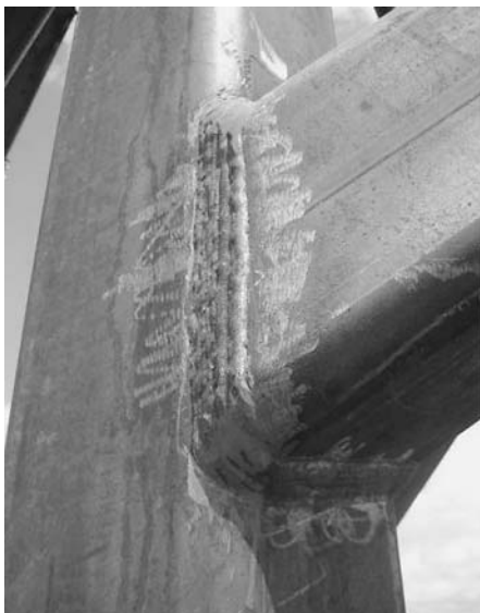
Figure 32. Welded connections for the reaction structure.
