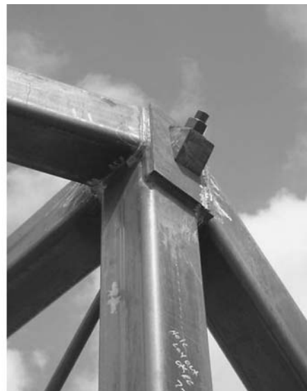
Figure 32. Welded connections for the reaction structure.
