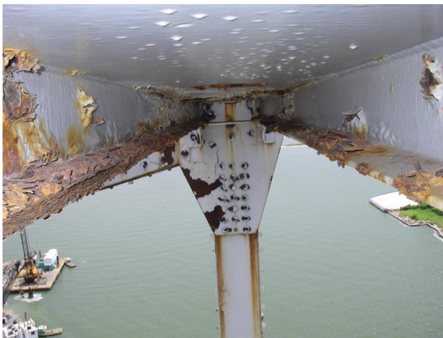
FIGURE 1.3.1 The underside of a steel bridge member exhibiting significant corrosion. Courtesy of the Texas Department of Transportation, © 2007. All rights reserved.
