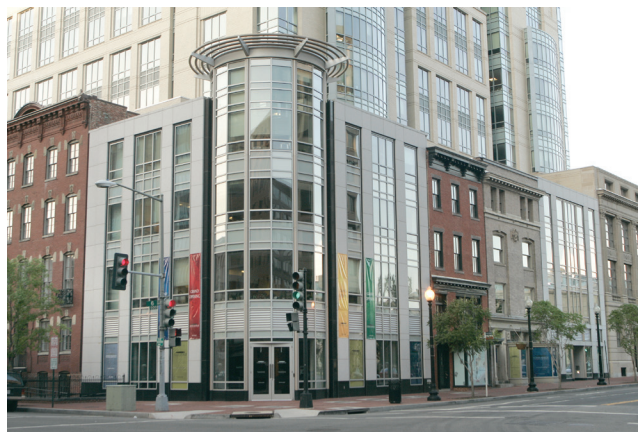
FIGURE 5-1 Marion Koshland Museum, located at the corner of 6th and E Streets, N.W., Washington, D.C. SOURCE: Marion Koshland Museum, 2010.
