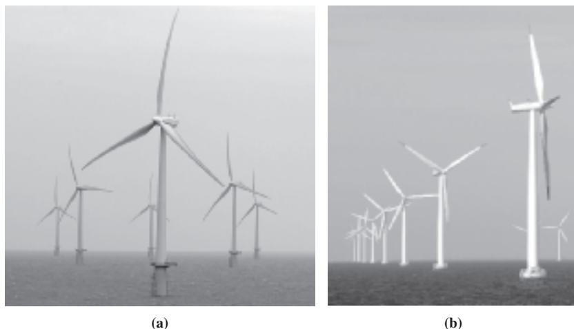
FIGURE 2-3 Common offshore wind turbines: (a) Vestas 3-MW turbines with 90-m rotor diameters and 70-m hub heights at Thanet in the United Kingdom. The turbines are on monopile foundations. (b) Siemens 2.3-MW turbines with 83-m rotor diameters and 69-m hub heights at Nysted off of Denmark. These turbines are on gravity-base foundations. (SOURCE: Vestas, Siemens.)
