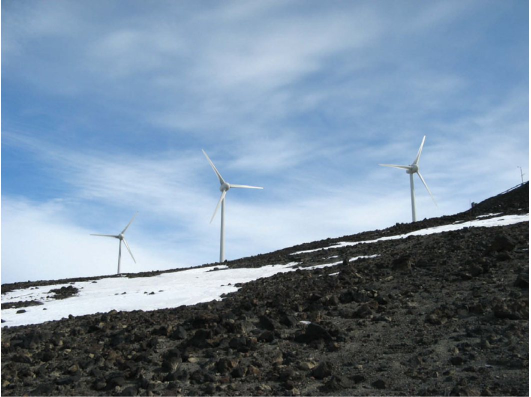
FIGURE 4.3 Three wind turbines located between McMurdo Station and Scott Base that provide energy to both stations. SOURCE: Mike Casey, NSF.
