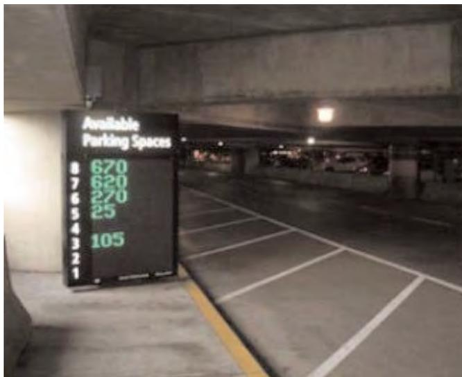
**Figure 4.16.** A parking availability sign that is placed immediately after the access controlled entrance plaza indicating to drivers the number of parking spaces available on each floor of the parking structure (SEA-TAC Airport). Note: Although the signage is useful and located in the correct location, if the information displayed is not current and accurate, drivers will soon discredit the information and the signage becomes useless.
