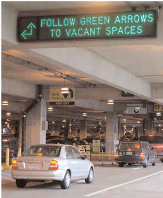
*Figure 4.18. The informational signage associated with a “space management system” that directs drivers to specific available parking spaces.*
