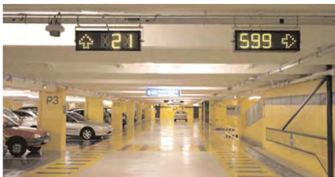
**Figure 4.19.** Once inside the parking garage, the space management system uses a series of signs to indicate which areas have available parking. Then sensors located above each parking space use red and green indicator lights to inform drivers if a particular space is occupied or not.
