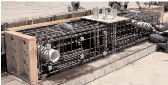
Figure 2.16. Reinforcing cage installed in form—HYB1.
