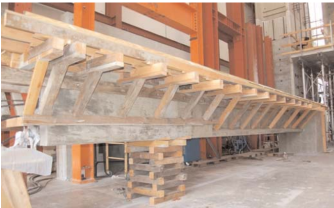
Figure 2.38. Construction of concrete deck reacting off girder.
