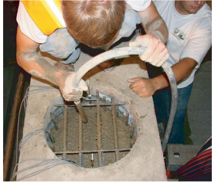
(b) Vibrating Concrete in Pocket
