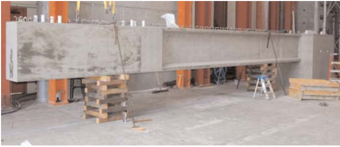
Figure 2.35. Girder on falsework prior to grouting closure joint.
