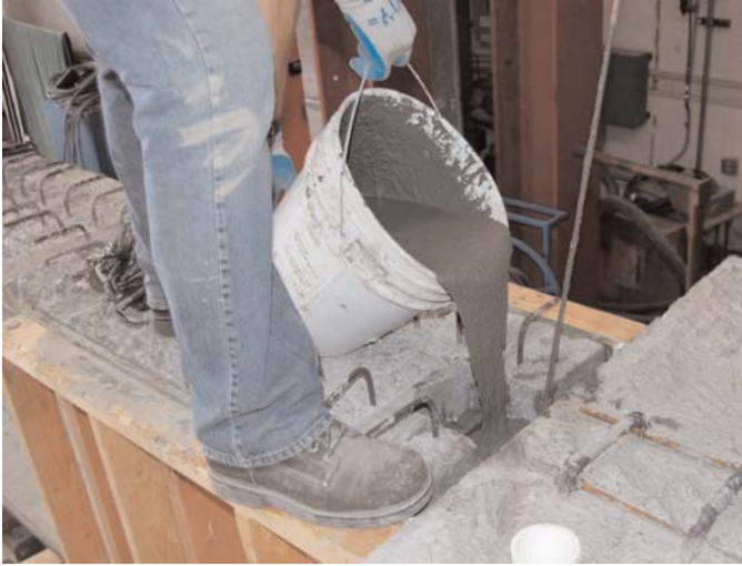
Figure 2.37. Grouting of girder to reaction block closure joint.
