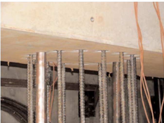
Figure 2.10. Cap placement during and after cap setting operation—GD.
