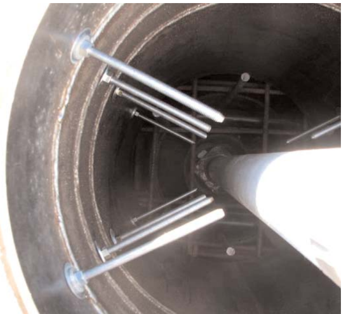
Figure 2.20. View inside steel shell showing weld beads—HYB2.
