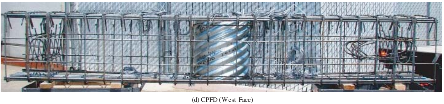
Figure 2.13. Comparison of cap pocket bent cap rebar cages during fabrication.
