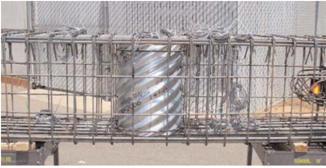
Figure 2.3. Rebar cage with corrugated pipe and supplementary hoops—CPFD.
