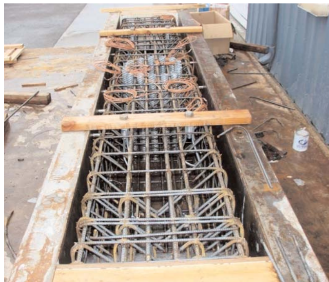
Figure 2.8. Bent cap rebar cage in form during fabrication—GD.
