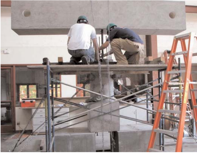
Figure 2.17. Bent cap setting operation—HYB1.
