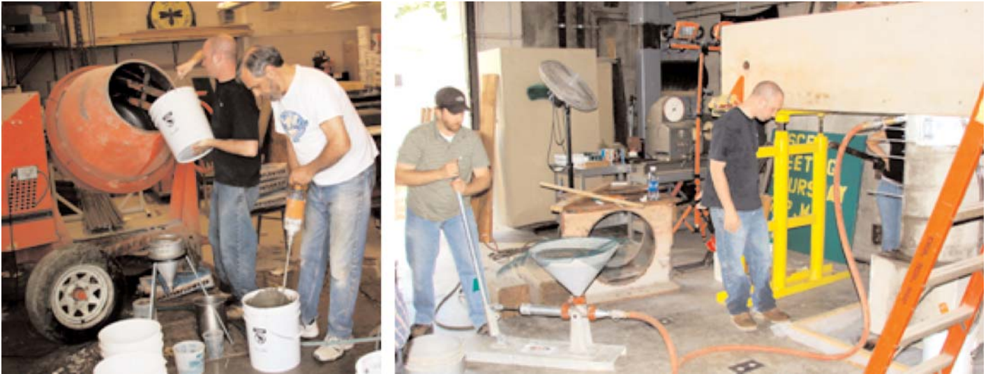
Figure 2.11. Mixing and pumping of grout—GD.
