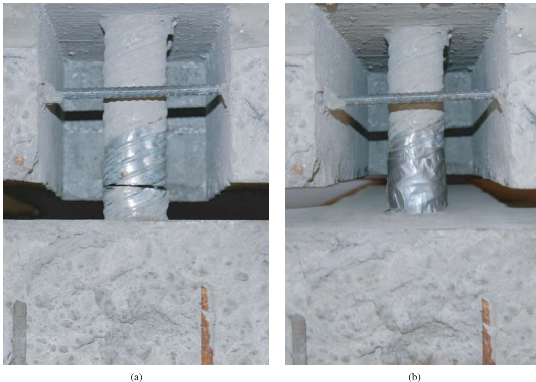
Figure 2.36. Girder post-tensioning duct (a) prior to splicing and (b) after splicing.
