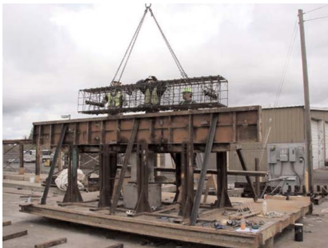
Figure 2.6. Lowering bent cap rebar cage into elevated formwork—CIP.
