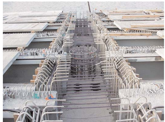
Figure 1.3. San Mateo-Hayward Bridge widening project (12).
