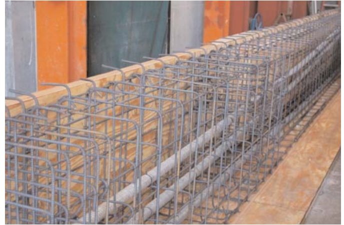
Figure 2.34. Girder reinforcing cage.
