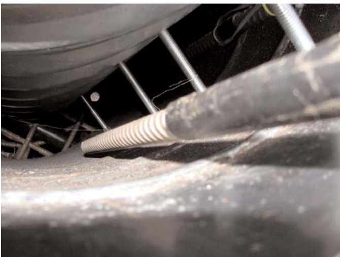
Figure 2.22. View down dual shell prior to casting with rebar—HYB3.
