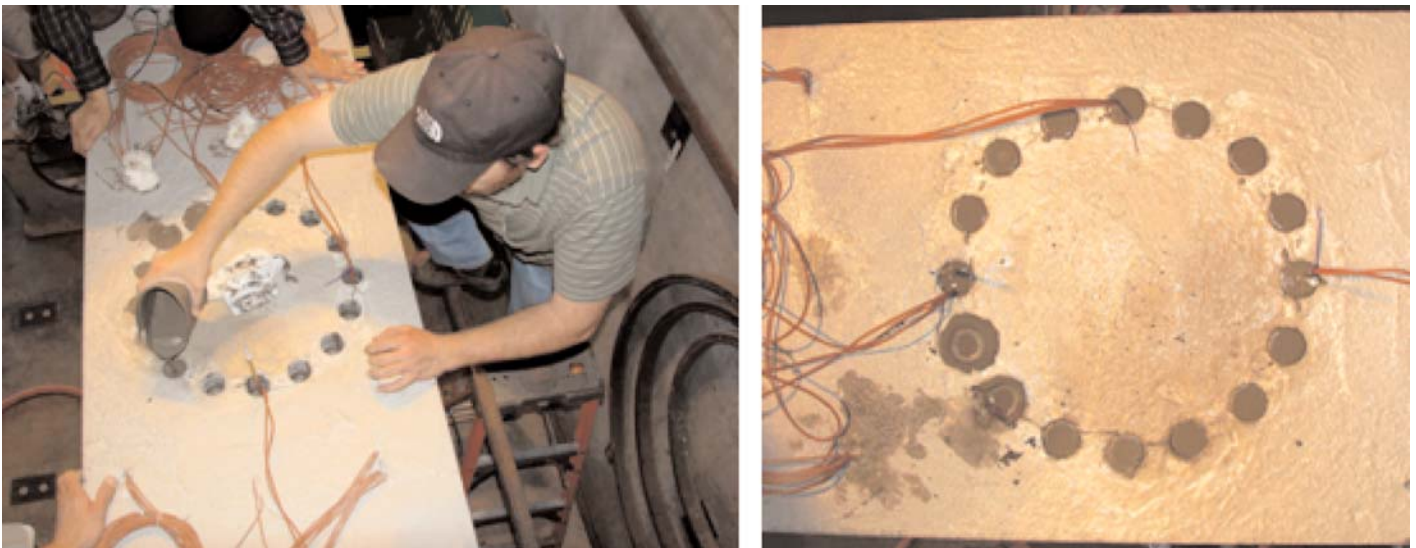
Figure 2.12. Topping off ducts with grout and cap top post-grouting—GD.
