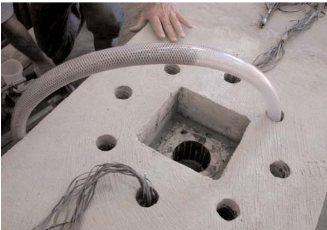
Figure 2.18. Bedding layer and corrugated duct grouting operation—HYB1.
