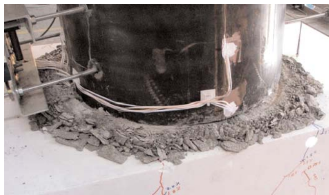
Figure 2.79. Bedding layer grout deterioration at end of test—HYB3.
