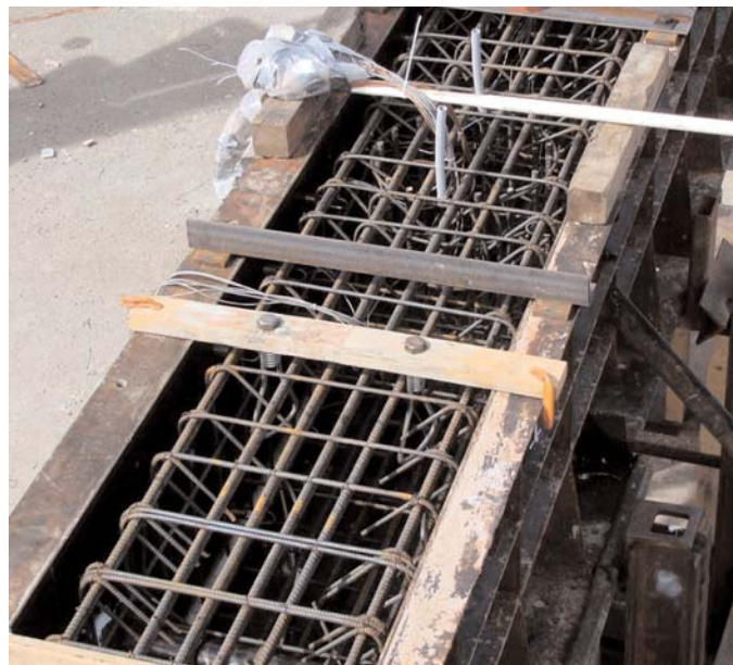
Figure 2.7. Bent cap rebar cage in form during fabrication—CIP.
