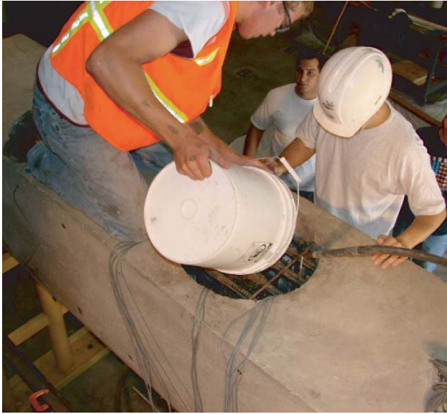
(a) Bucketing Concrete into Pocket
