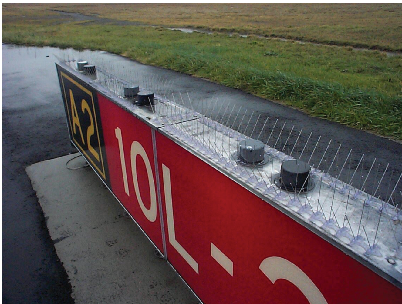
FIGURE 11 Antiperching devices used to deter birds from a low level windshear alert system (Source: Steve Osmek).
