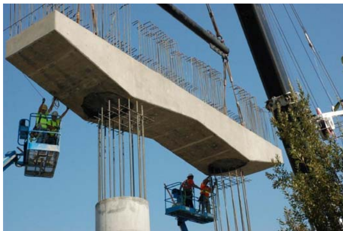
Figure 9. Grouted duct lower stage cap erection (Washington State DOT SR 520/SR 202).
