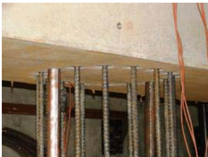
Figure 8. Grouted duct cap construction and cap placement (Matsumoto 2009b).
