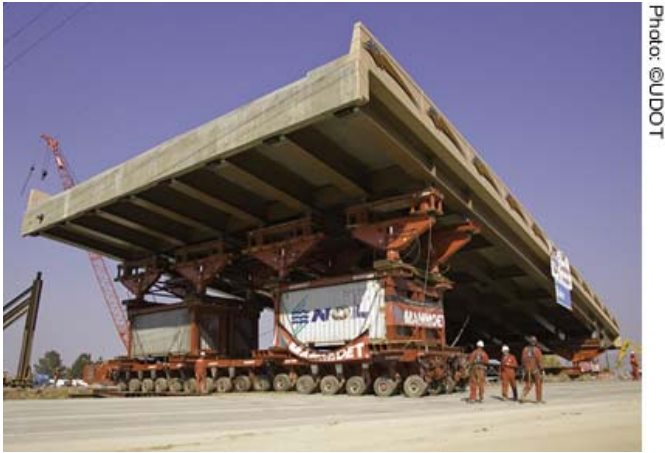
Figure 21. Prefabricated superstructure installed using SPMTs (Utah DOT).
