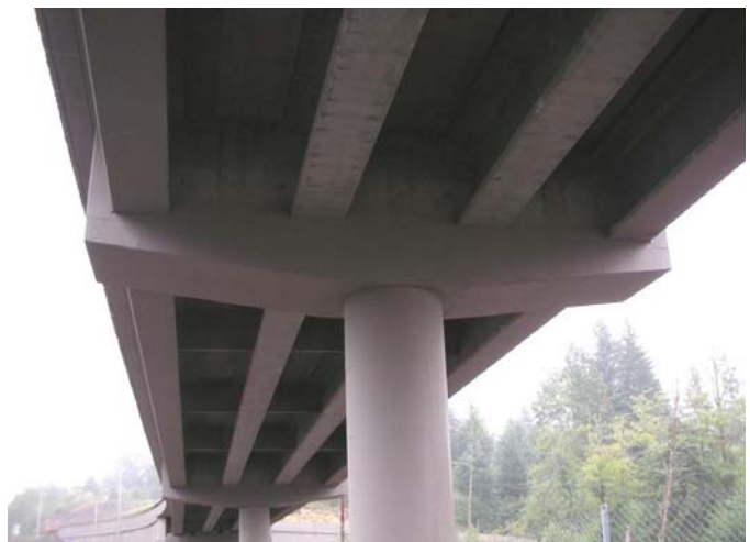
Figure 14. Two-stage cap beam with prestressed girders.
