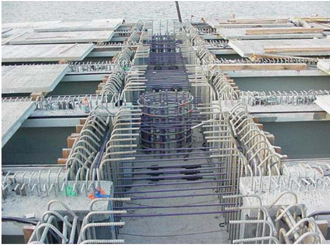
Figure 15. Integral precast lower stage cap with precast girders (Restrepo, Matsumoto, and Tobolski 2011).
