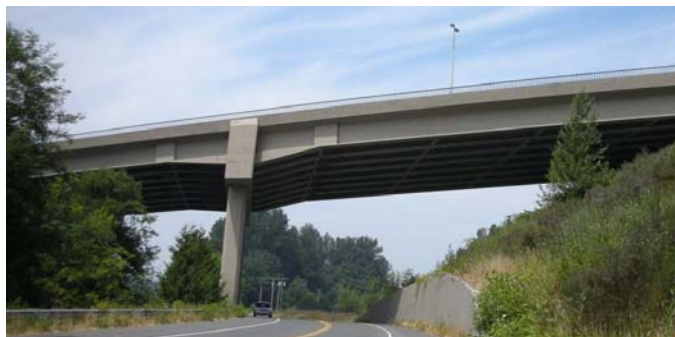
Figure 26. Spliced girder bridge with precast pier segment (BergerABAM).
