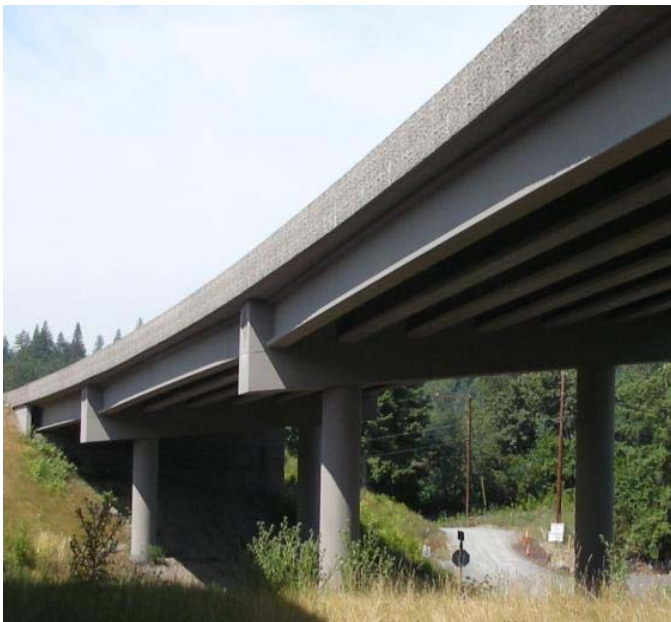
Figure 23. Typical precast, prestressed girder bridge in Washington State.
