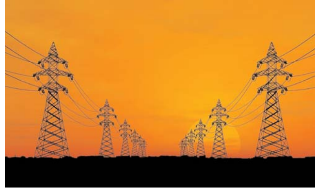
FIGURE 7 Transmission lines at sunset ( courtesy: HMMH ).
