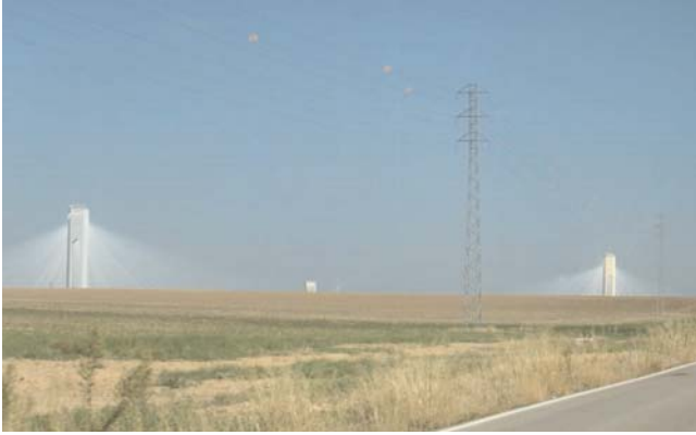
FIGURE 22 Power Tower Abengoa Energy, Spain ( courtesy: Dr. Clifford Ho, U.S. DOE, Sandia National Laboratories).
