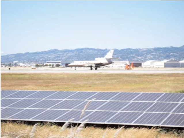
FIGURE 13 Solar PV at Oakland International Airport, California (courtesy: HMMH).
