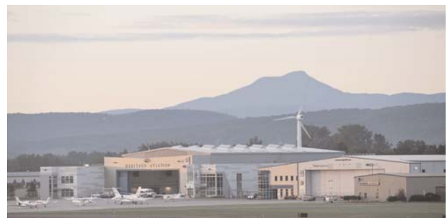
FIGURE 18 Wind turbine at Burlington International Airport, Vermont (courtesy: Christopher Hill, Heritage Aviation).
