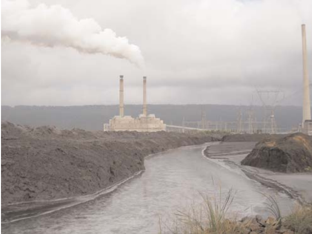
FIGURE 6 Power plant ( courtesy: U.S. EPA website ).
