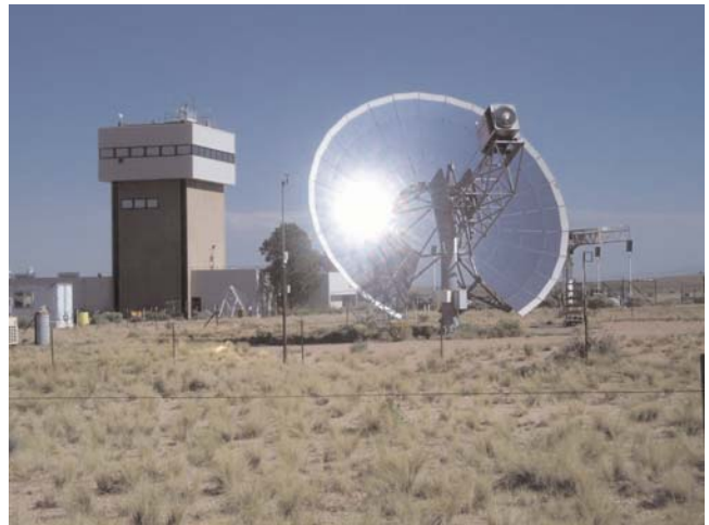
FIGURE 4 Dish Stirling at Sandia National Laboratories (courtesy: Dr. Clifford Ho, U.S. DOE, Sandia National Laboratories).
