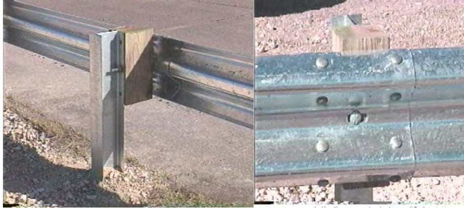
Figure 50. Modified G4(1S) guardrail with routed wood blockouts.
