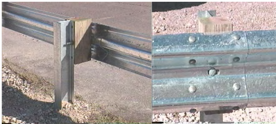
Figure C6-1: Modified G4(1S) guardrail with routed wood blockouts
