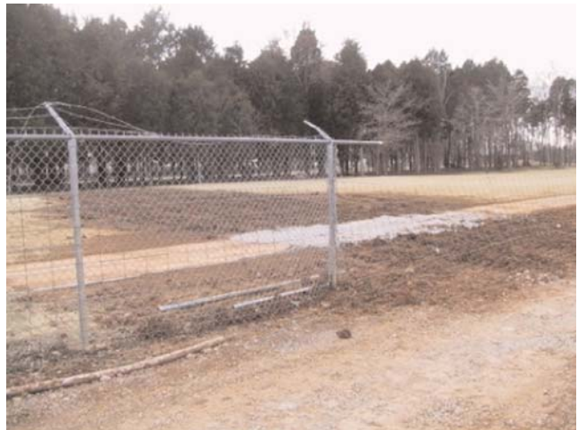
FIGURE 34 Downed fencing. Used with permission.
