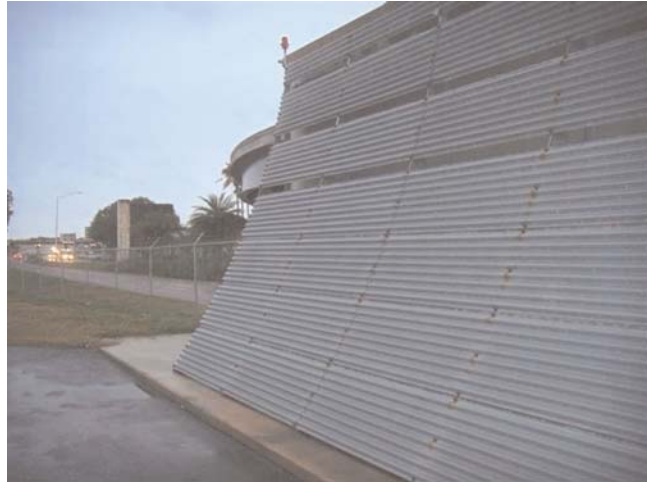
FIGURE 33 Blast fence. Source: F. Dettmann, A.A.E., Hillsborough County Aviation Authority, Tampa International Airport.
