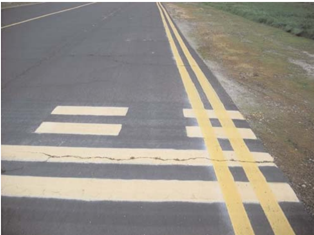
FIGURE 18 Incorrect marking precedence. Source: Lammerding 2010b.
