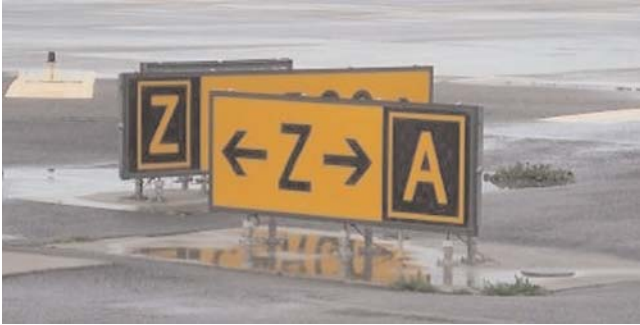
FIGURE 21 Reversed signage. Source: Lammerding 2010b.
