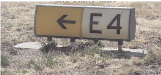
FIGURE 22 Faded sign panel. Source: Lammerding 2009.
