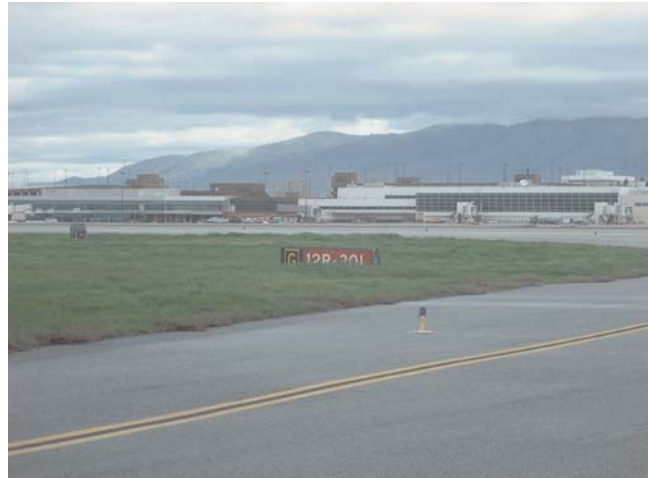
FIGURE 20 Sign obscured by vegetation. Source: Lammerding 2010a.
