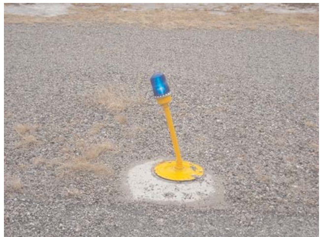
FIGURE 24 Bent taxiway edge light. Source: P. Khera, Alaska DOT.
