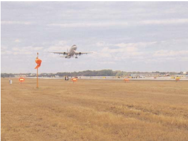
FIGURE 25 Wind sock and Precision Approach Path Indicators in operation. Source: F. Dettmann, A.A.E., Hillsborough County Aviation Authority, Tampa International Airport.
