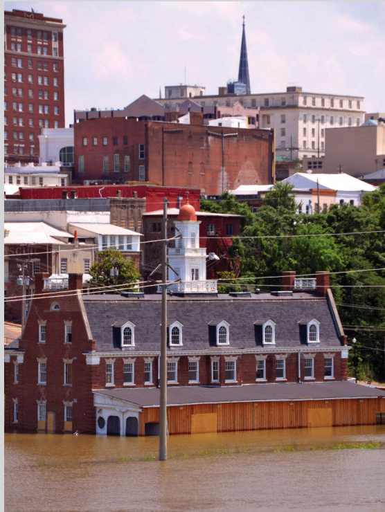
Train depot flooded by the Mississippi River, Vicksburg, Mississippi, May 13, 2011.
