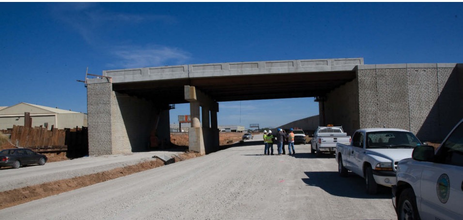
Phased construction for Pennsylvania Avenue over the Union Pacific Railroad.
