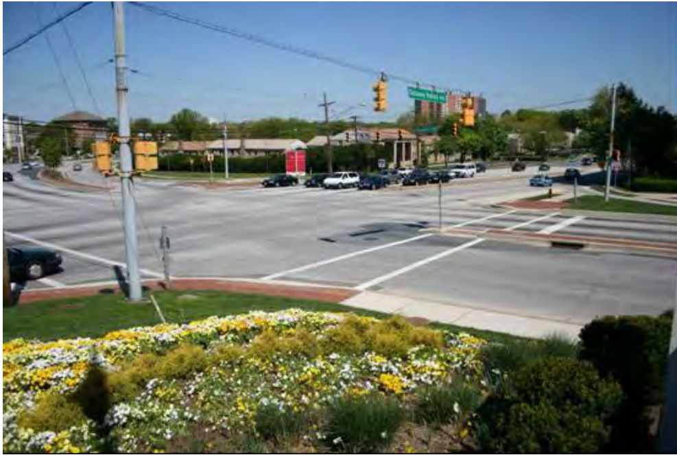
Figure 33. Dulaney Valley Road/Fairmount Avenue, Towson, MD
