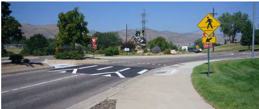
Exhibit 6: South-East Quadrant – View of Raised Crosswalk
