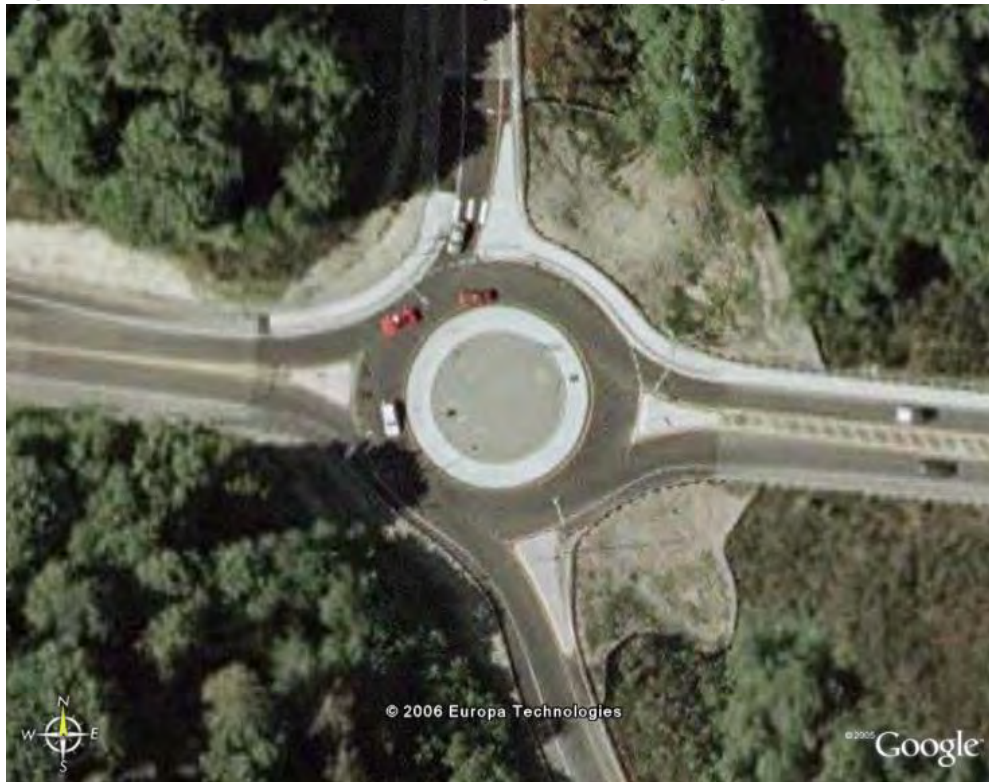
Figure 28. WA 16 Southbound/Borgen Boulevard, Gig Harbor, WA
