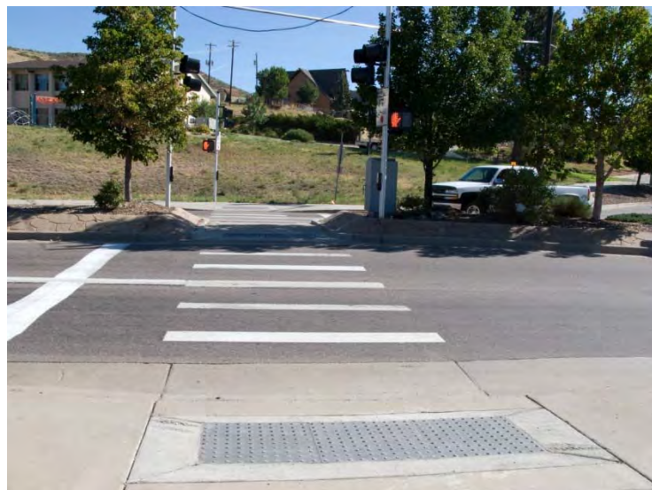
Exhibit 10 - Two stage, signalized pedestrian crossing
