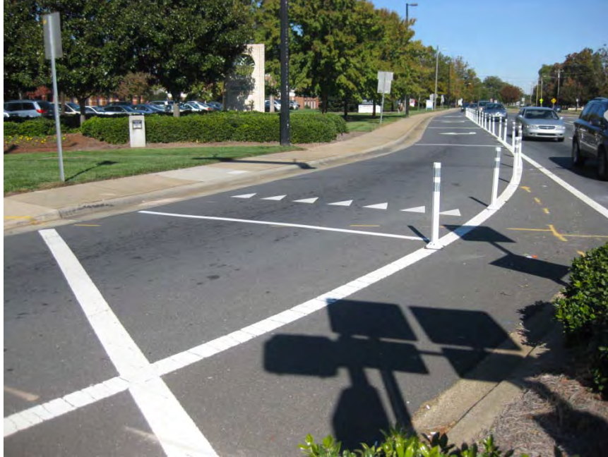
Exhibit 2: North-west Quadrant - View of Sound Strips and Lane Delineators
