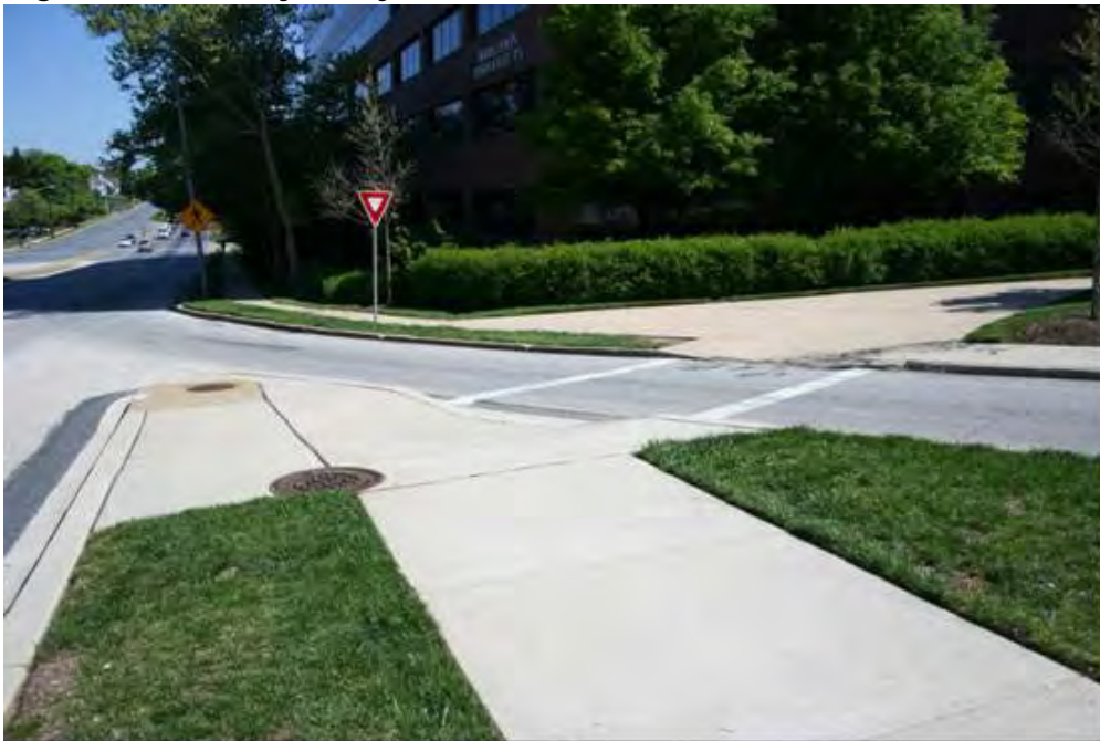
Figure 34. Dulaney Valley Road/Fairmount Avenue, Towson, MD
