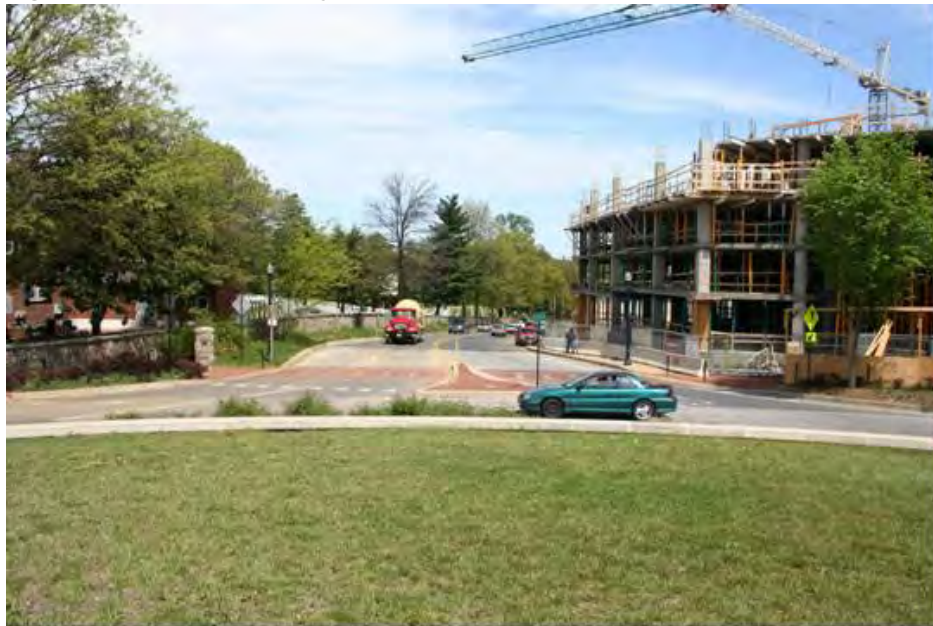
Figure 10. Spa Road/Taylor Avenue, Annapolis, MD
