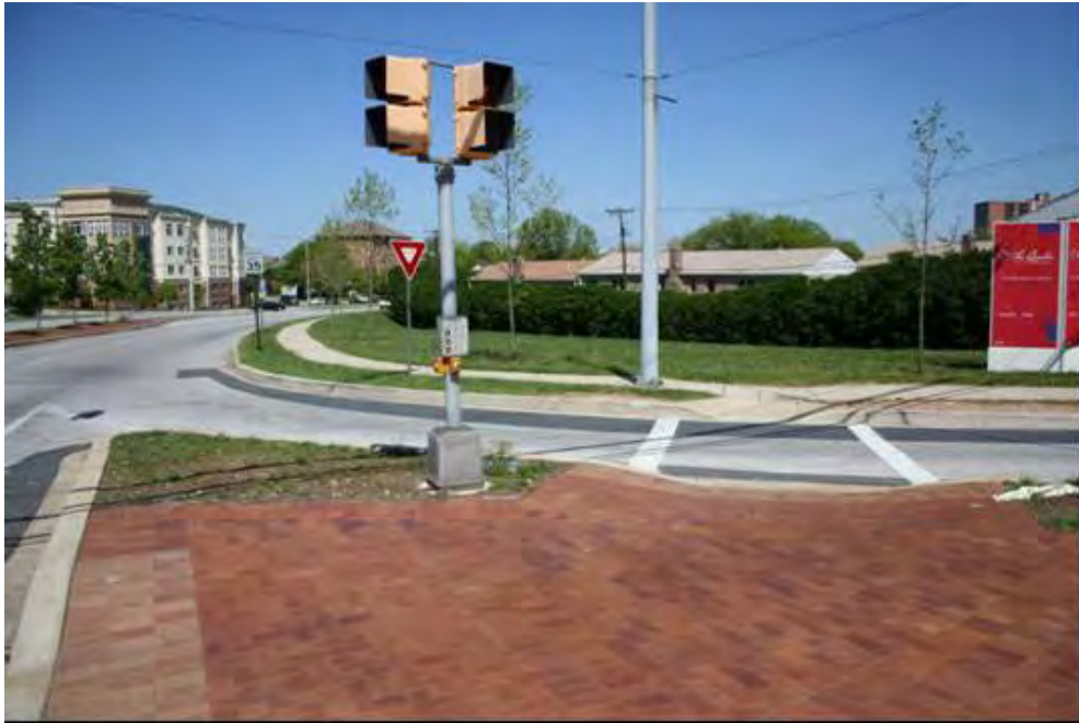
Figure 35. Dulaney Valley Road/Fairmount Avenue, Towson, MD
