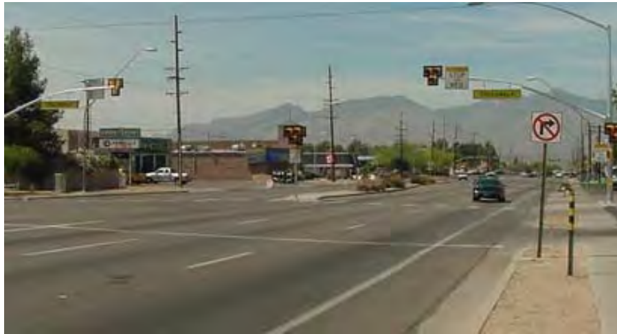
Exhibit 8 – Pedestrian Hybrid Beacon – Note the reverse dog-house signal head that houses the two red indications and the yellow indication. The two lenses at the top of the signal head are red and flash back and forth during the clearance interval. The yellow lens is located on the bottom of the signal head. (Tucson, DOT)
