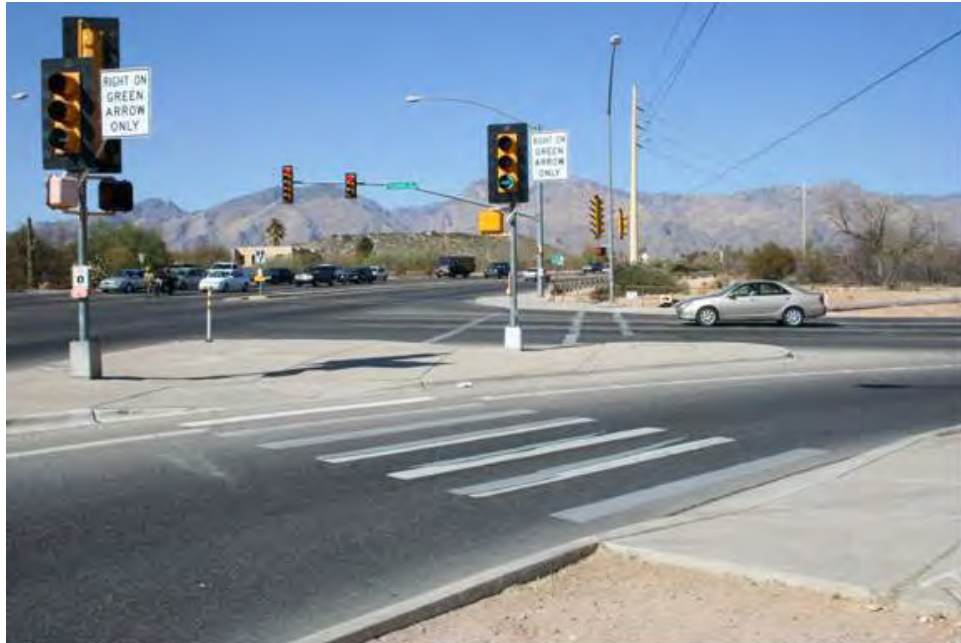
Figure 39. Sabino Canyon Road/Cloud Road, Tucson, AZ
