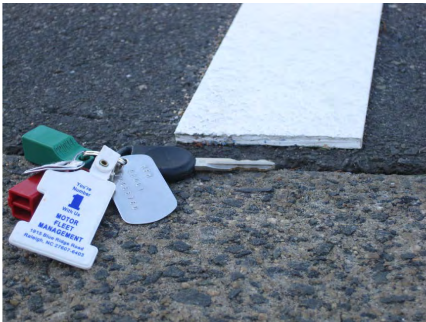
Exhibit 3: Close-Up View of Sound Strip Profile
