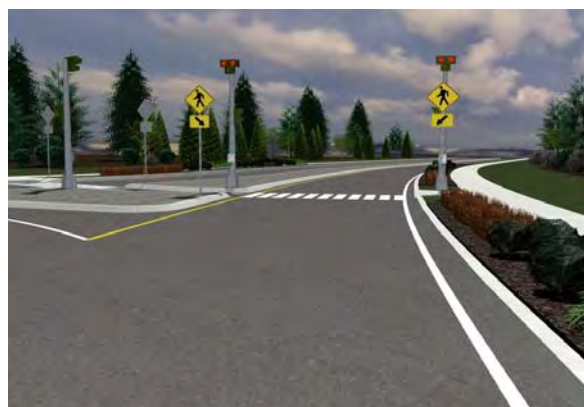
Figure 8. Driver View Approaching Exit Lane With HAWK Signal
