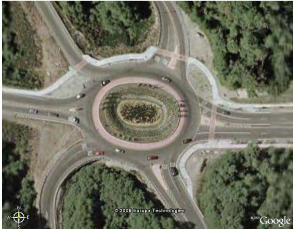
Figure 18. WA 16 Northbound/Borgen Boulevard, Gig Harbor, WA
