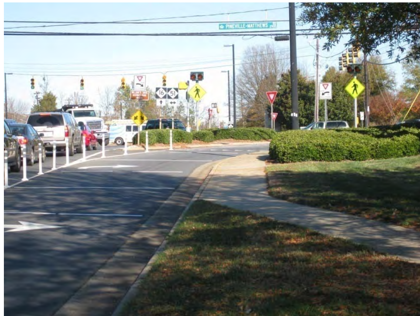
Exhibit 4: South-East Quadrant - View of Sound Strips, Delineators, and Flashing Beacons
