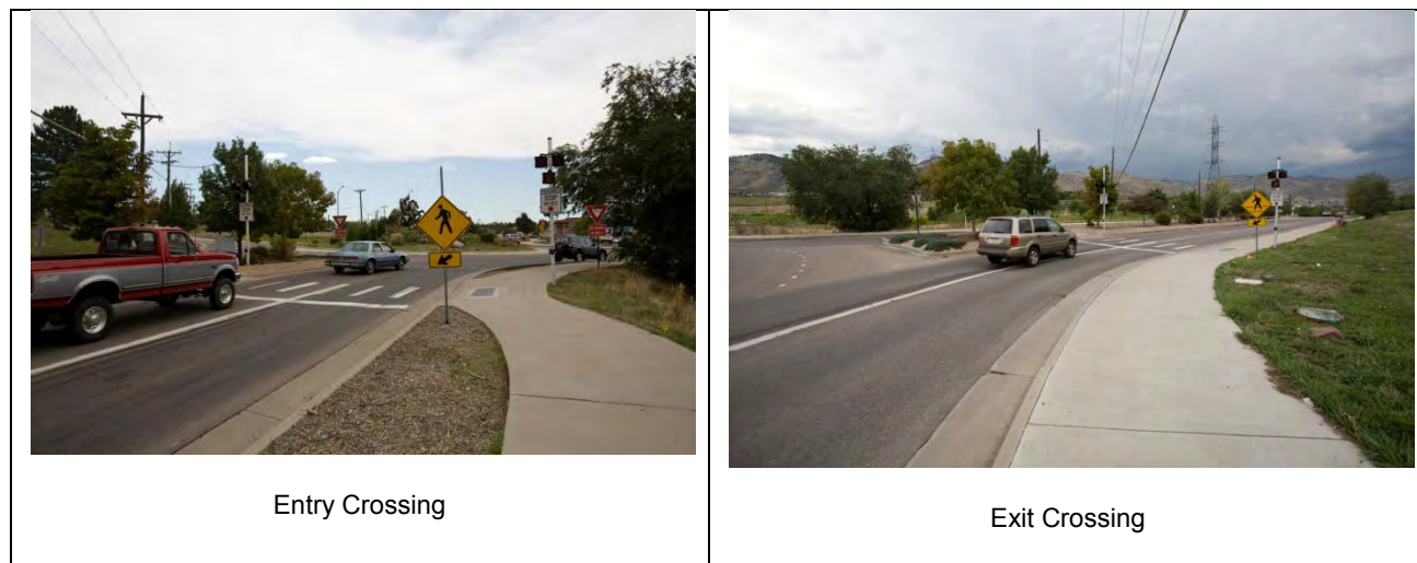
Exhibit 9 – HAWK signal test site following installation
