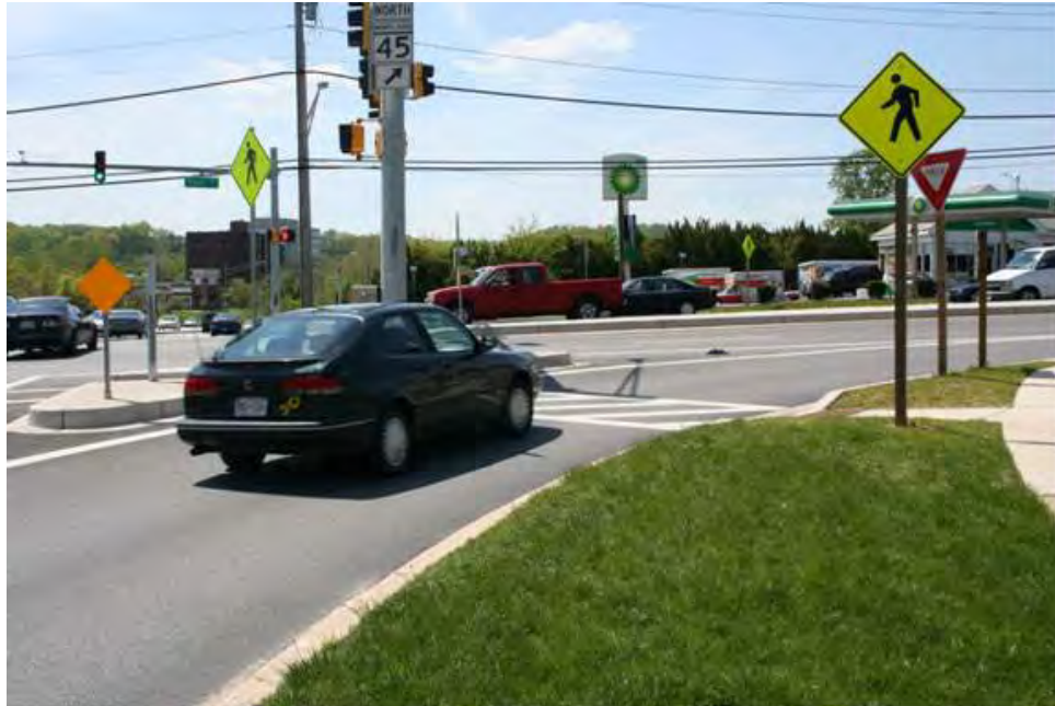
Figure 37. Padonia Road/York Road, Timonium, MD
