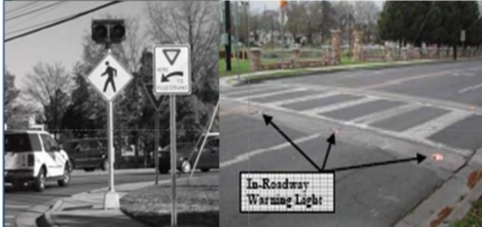
Exhibit 3 – Active When Present Flasher and In-Roadway Flashers (Fitzpatrick et al., 2006)
