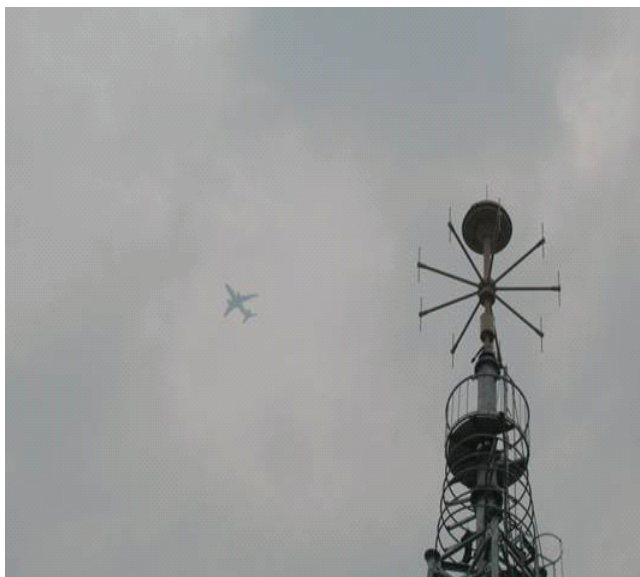
FIGURE 10 Fixed radio monitoring stations. Source: Beijing Radio Administration Bureau, at http://www.bjrab.gov.cn/jcjc/jcs/twzs/20101221/368.shtml .
