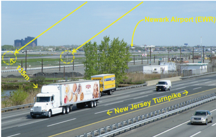
FIGURE 5 In harm's way—FAA GBAS installation at EWR.
