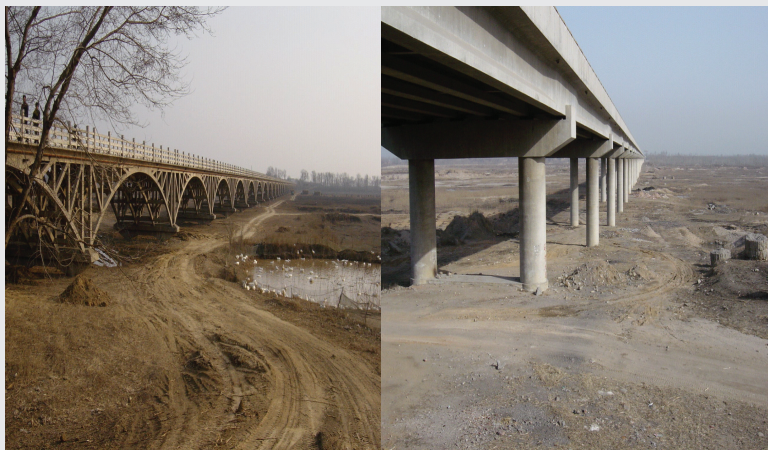
FIGURE 2-4 Eco-environmental consequences of groundwater depletion in China: a bridge over a dried-up river (left); former riverbed used for farming (right). SOURCE: Photos courtesy of Chunmiao Zheng, University of Alabama.
