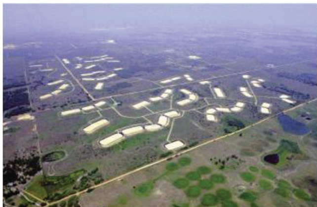
FIGURE 2-5 Rapid infiltration basins at the Water CONSERV II facility in Orlando, Florida, which recharged 31 MGD (120,000 m 3 /d) of reclaimed water in 2006. SOURCE: Alley et al. (1999).
