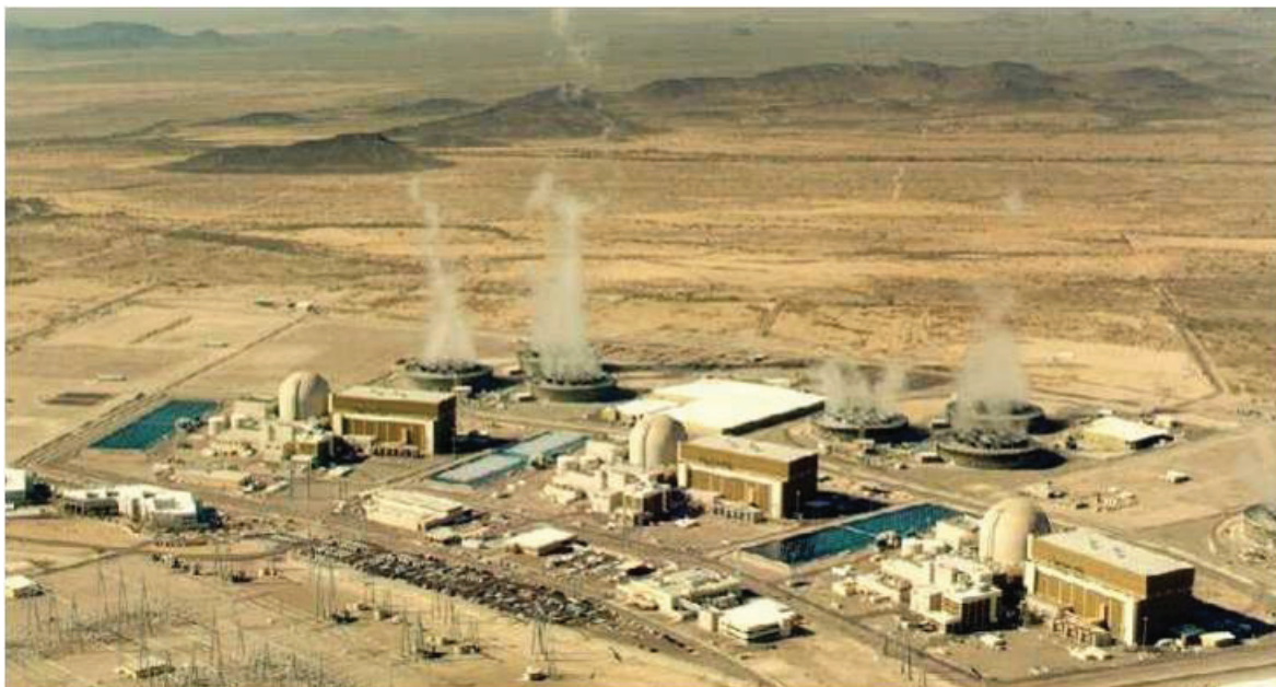
Palo Verde Nuclear Generating Station. SOURCE: Photo courtesy of Henry Day.
