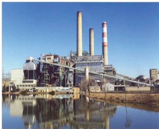
The Xcel Energy Cherokee Station. SOURCE: Photo courtesy of Xcel Energy ( www.XcelEnergy.com )
