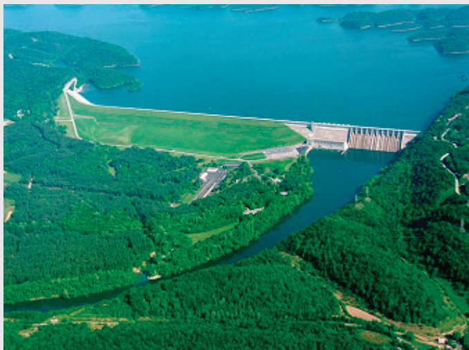
FIGURE 1 Wolf Creek Dam on the Cumberland River in Kentucky. SOURCE: USACE, Nashville District, 2011.
