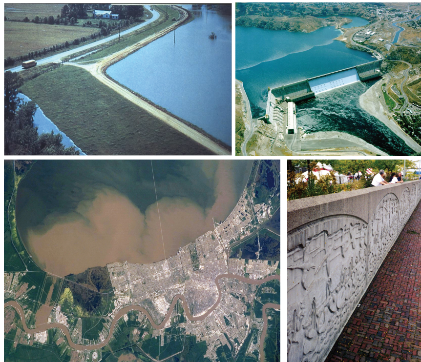
FIGURE 2.4 Structural Flood Mitigation Measures, clockwise from top left: Mississippi River levee; Grand Coulee Dam on the Columbia River in Washington; a floodwall that protects the city Winona, Minnesota, along the Mississippi River; and the Bonnet Carré Spillway, a floodway that diverts water from the Mississippi River into Lake Ponchartrain to reduce the flow passing New Orleans.
