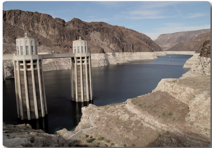
Water demands from Las Vegas, Nevada, combined with years of below average precipitation have drained Lake Mead to record-low levels, leaving a white “bathtub ring” 100 feet high.
