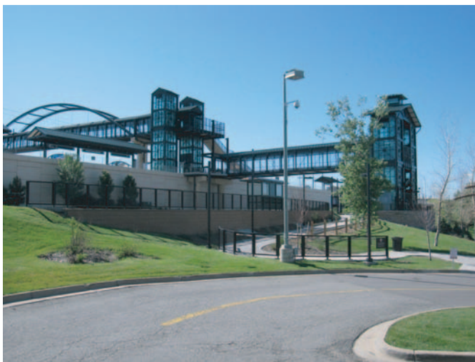
Exhibit 7-2. Pedestrian ramp providing station access (County Line RTD Station, Englewood, CO).
