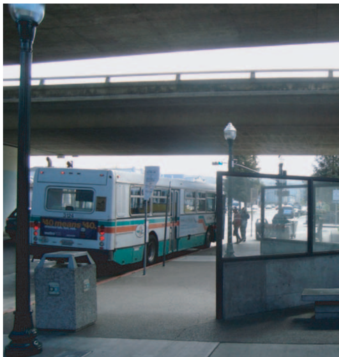
Exhibit 9-4. On-street bus facility example (Oakland, CA).
