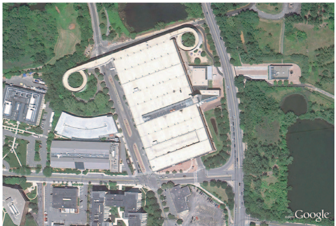
Exhibit 10-16. Bus access around parking structure (Cambridge, Massachusetts).
