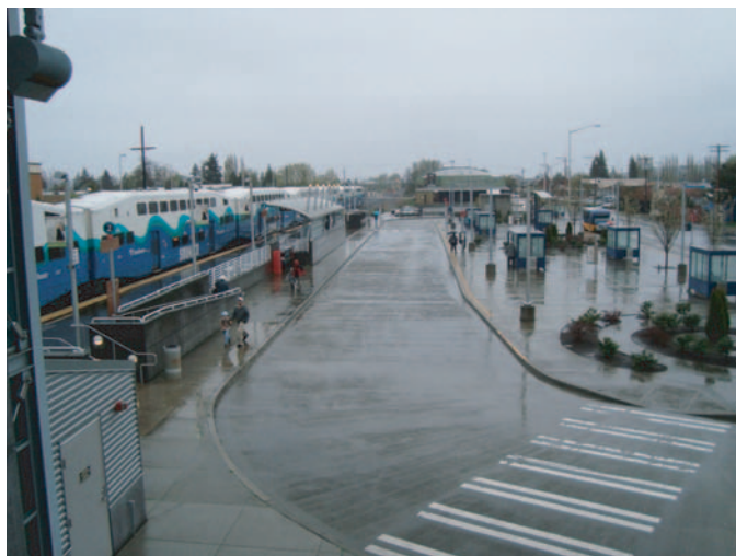
Exhibit 9-3. Feeder bus connections located close to station platform (Sound Transit Commuter Rail Station, Kent, WA).
