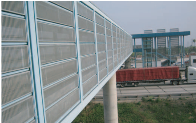
Exhibit 4-1. Footbridge providing access to Sierra Madre Station, CA.
