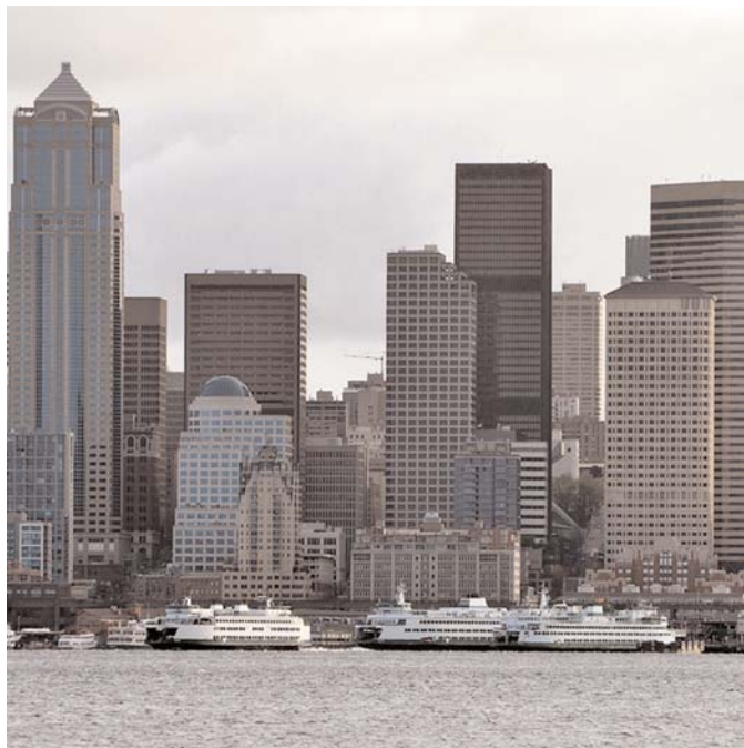
Figure 5-13. Washington State Ferry—downtown Seattle terminal.
