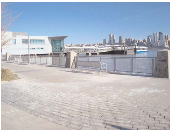
Figure 5-4. New York Waterway Weehawken Terminal.
