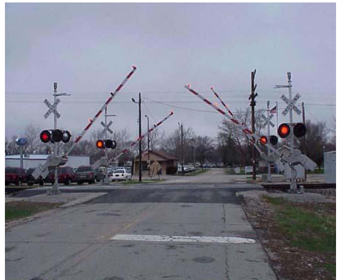
Figure 8-1. Four-quadrant gate grade crossing treatment in Gardner, Illinois (U.S. Department of Transportation 2008b).
