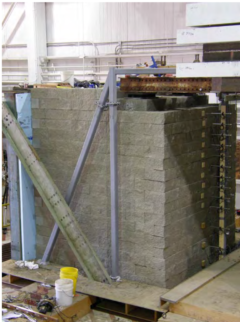
Figure 5.7: Completed GRS Abutment with the Bridge
