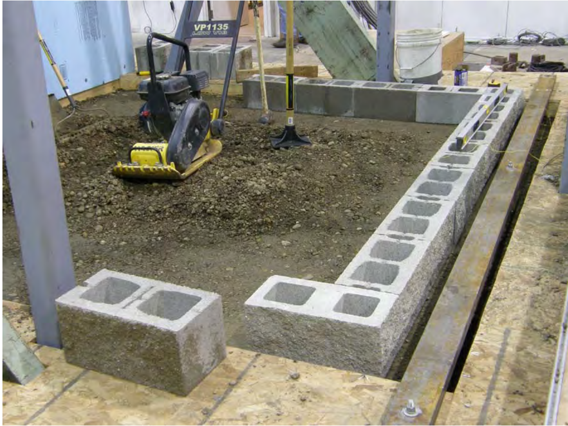
Figure 5.5: First Course of Block Placement
