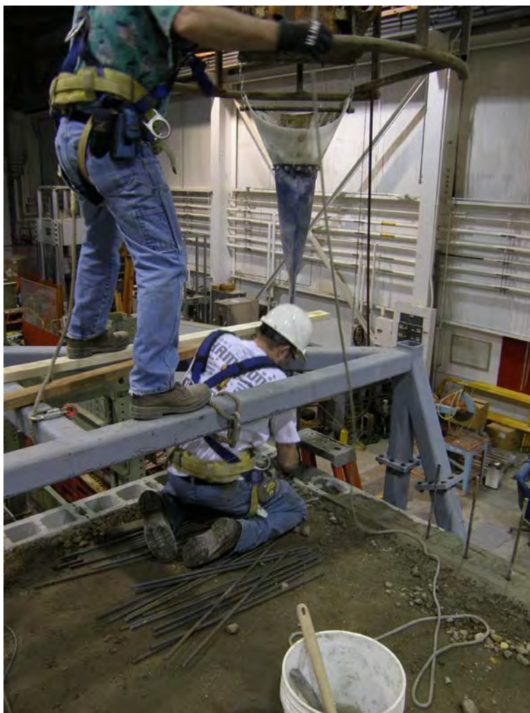
Figure 5.6: Grouting the Top Three Courses of Blocks
