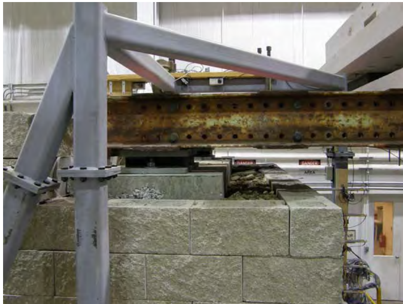
Figure 6.11: Photograph of Abutment Sill Movement after 1.0 g Test at 3 Hz
