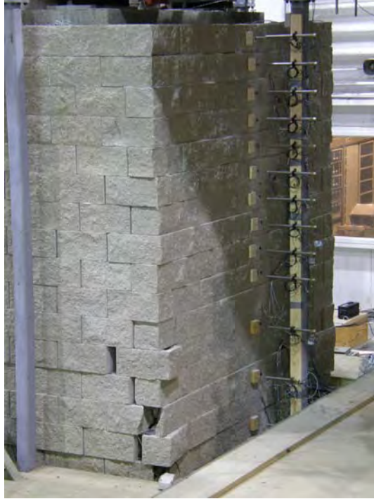
Figure 6.8: Photograph of Block Damage after 1.0 g Test at 3 Hz
