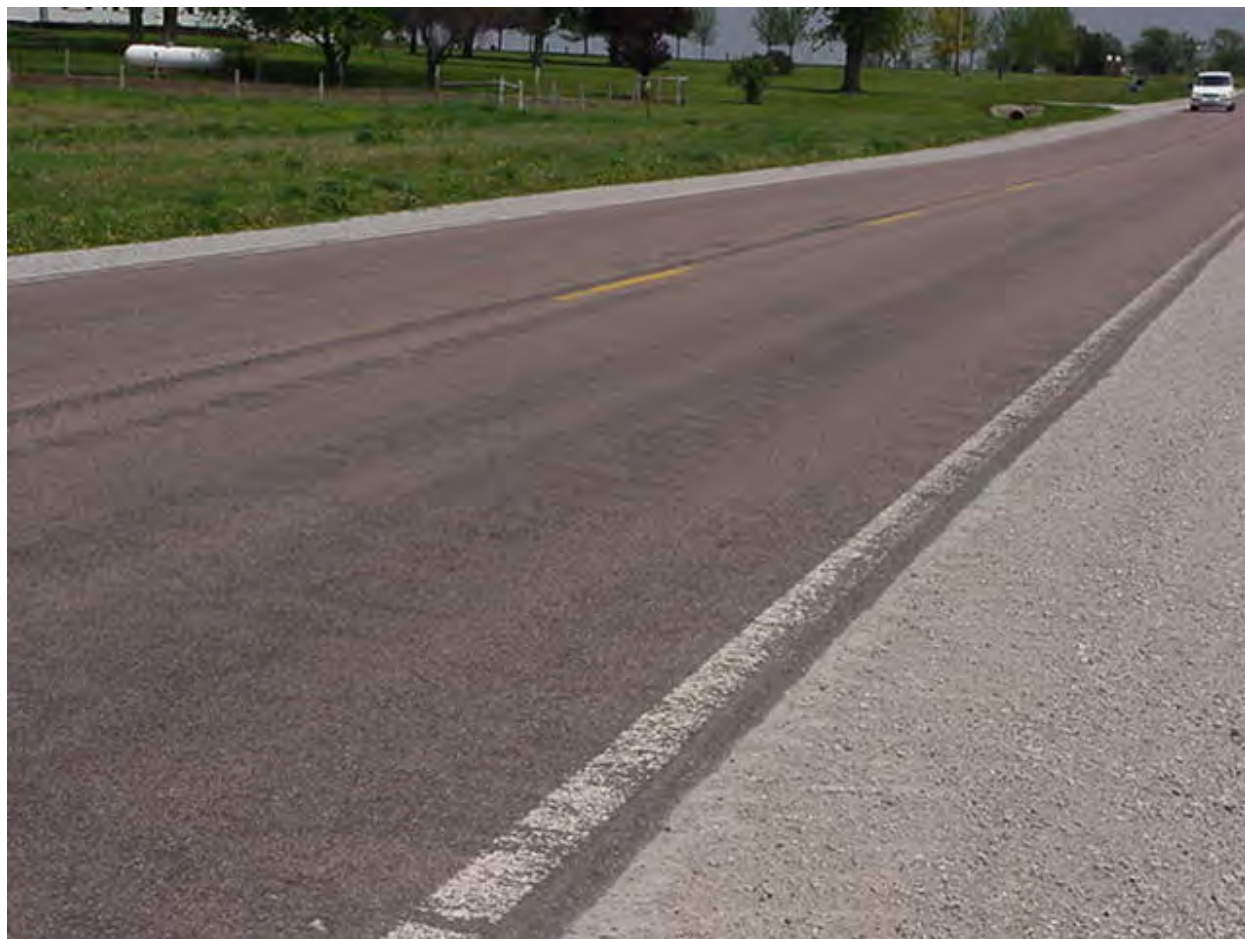
FIGURE 2 Highway 927 in Iowa, from May 2000, showing chatter markings from plowing subsequent to a microsurface treatment in 1999.
