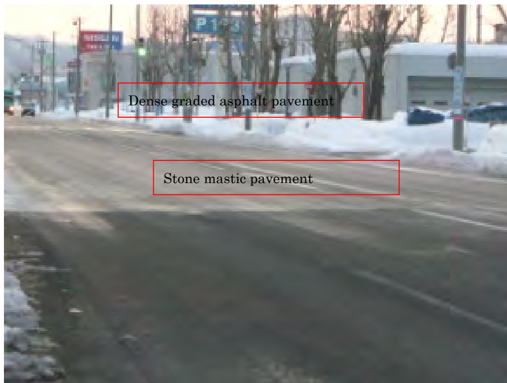
FIGURE 2 Difference of road surface by pavement type
