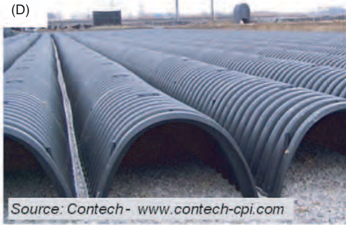
Figure 4.17. Examples of infiltration retrofits: (A) infiltration basin; (B) infiltration trench; (C) dry well; (D) proprietary underground infiltration systems.
