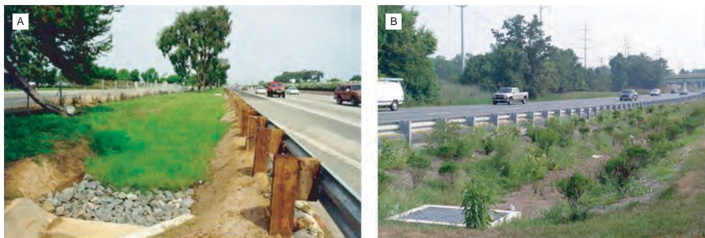
Figure 4.16. Two examples of vegetated filtration BMPs: (A) Caltrans grass-lined swale; (B) DelDOT bioretention area. Notice siting along narrow landscape strips behind guardrails.
