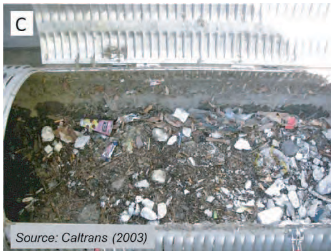
Figure 7.1. Four examples of BMP conditions requiring maintenance: (A) excessive accumulation of sediments in underground detention; (B) clogged pipe; (C) accumulation of trash and debris in a GSRD; and (D) excessive vegetation near an outlet.
