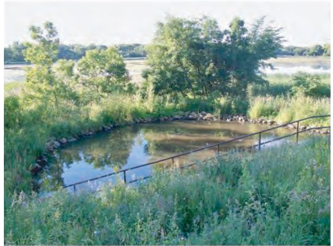
Figure 10.26. MnDOT I-35 retrofit, treatment forebay to Diamond Lake.
