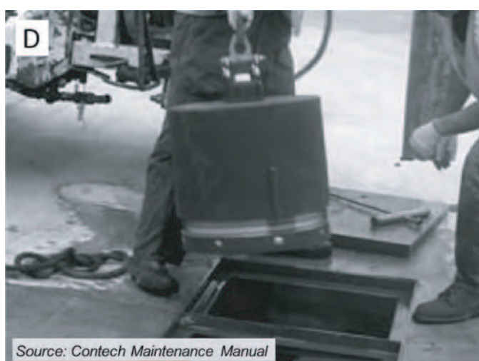
Figure 7.2. Four examples of BMP maintenance activities: (A) vactoring solids from underground sumps; (B) removing sediments from surface BMPs; (C) replacing media in filtration BMPs; (D) replacing proprietary media cartridges.
