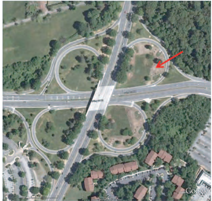
Figure 10.28. DDOT interchange retrofit project, aerial view.
