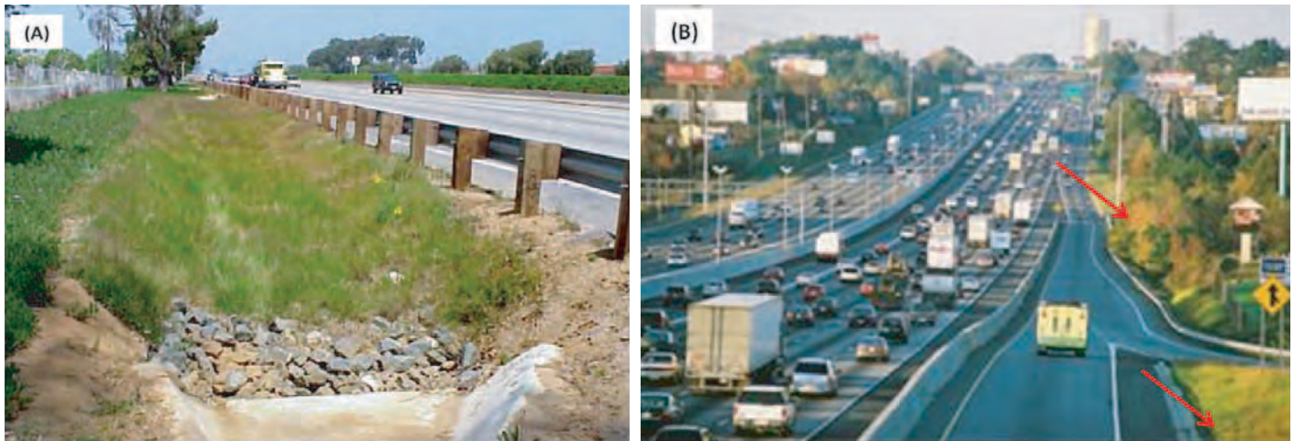
Figure 9.4. Highway surface conveyances: (A) Caltrans retrofit of a ROW strip adjacent to I-5 with a vegetated biofiltration swale and (B) roadside ditches adjacent to ramps, Atlanta, Georgia.
