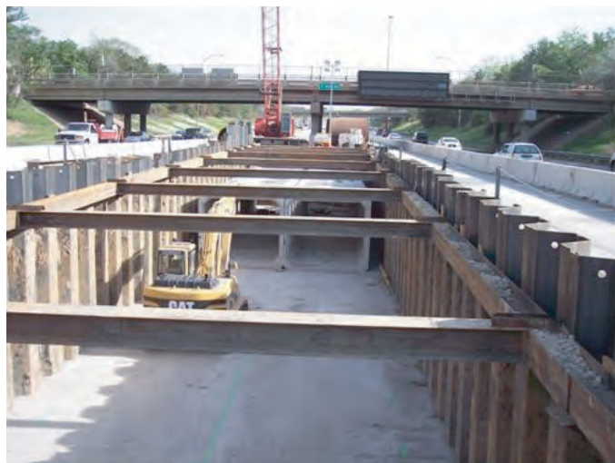
Figure 10.27. MnDOT I-35 retrofit, storm tunnel surge chamber construction.
