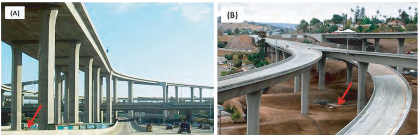
Figure 9.3. Two examples of vacant areas below elevated highway sections: (A) I-405/I-105 interchange, Los Angeles, and (B) dry extended-detention basin beneath SR-125/SR-94 interchange, San Diego County.
