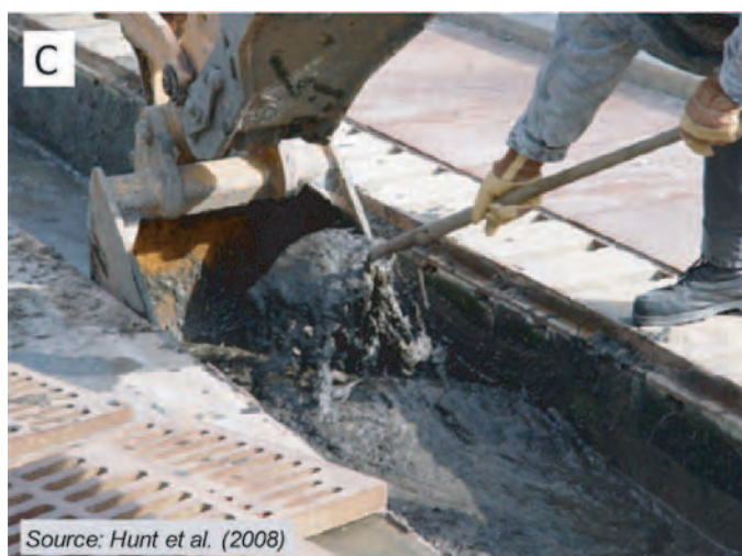
Figure 7.2. Four examples of BMP maintenance activities: (A) vactoring solids from underground sumps; (B) removing sediments from surface BMPs; (C) replacing media in filtration BMPs; (D) replacing proprietary media cartridges.
