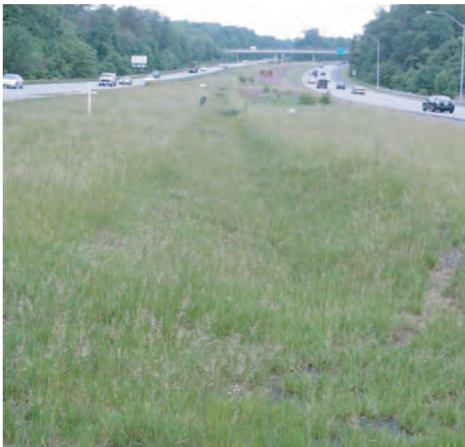
Figure 10.35. Standard swale design in the media with adjacent minimal filter strip (left); modified narrow swale design without filter strip (right).
