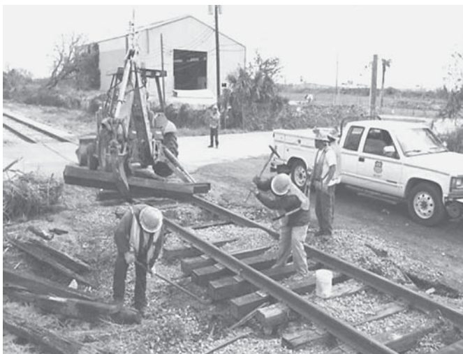
Figure 5-7. Rail repairs on Galveston Island, Texas.
