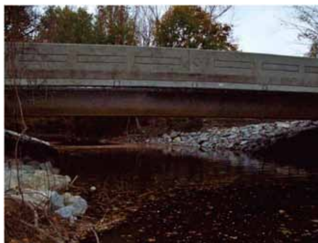
FIGURE 17 Finished 981G Ramapo River Bridge (Courtesy NYSDOT).
