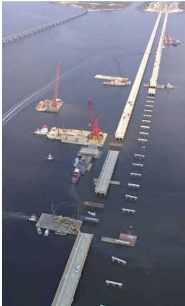
FIGURE 5 I-10 Escambia Bay Bridge repairs in progress (Courtesy FDOT).
