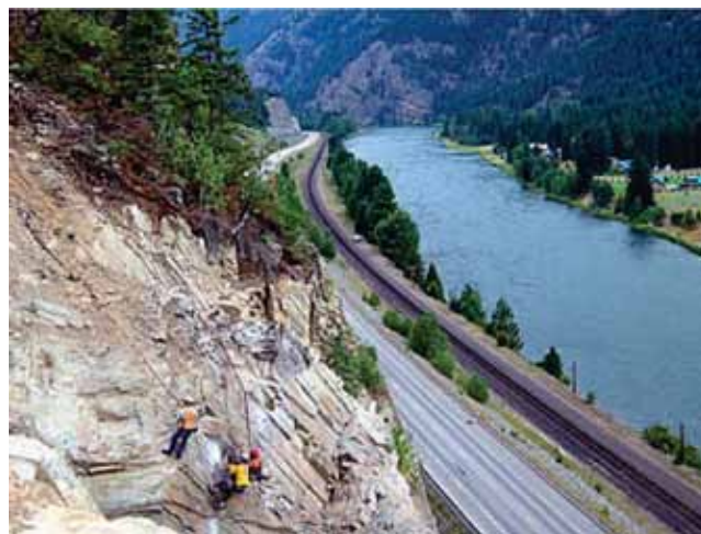
FIGURE 13 Scaling operations on US-2.
