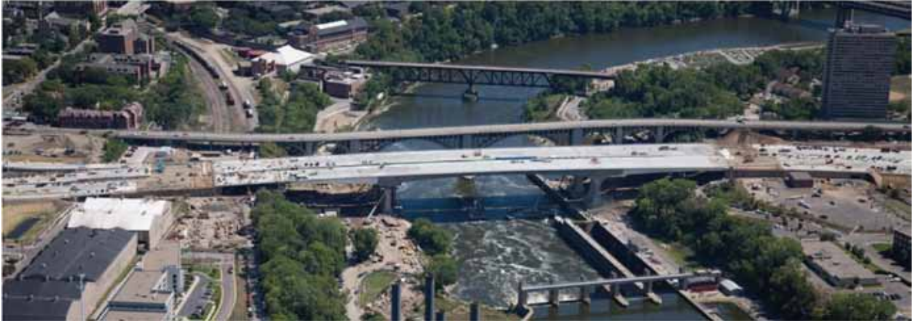
FIGURE 10 Completed I-35W St. Anthony Falls Bridge.
