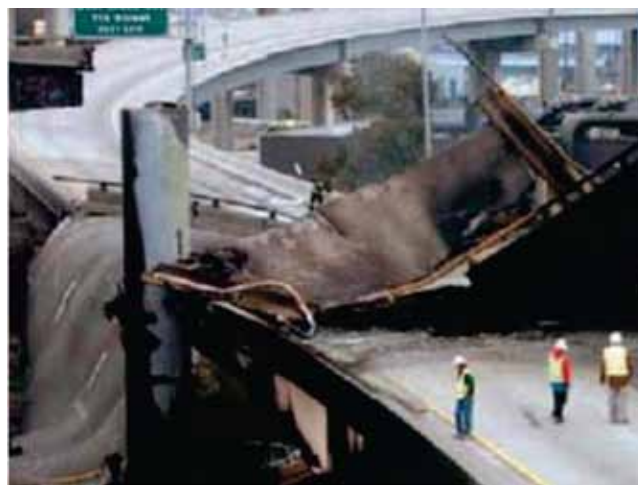
FIGURE 4 I-580/880 accident and fire aftermath (Blanchard et al. 2009).
