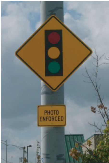
Figure H-9. Advance warning sign for red light camera enforced intersection.
