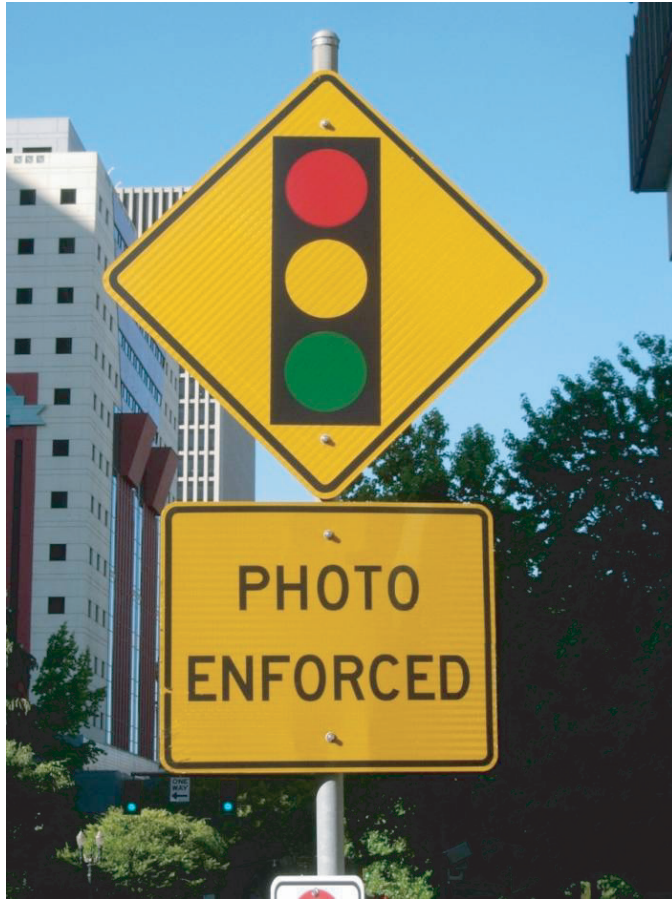
Figure H-6. Advance warning sign for red light camera enforced intersection.
