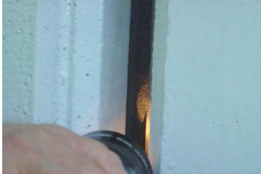
Photo 5. Filter fabric visible in joint
