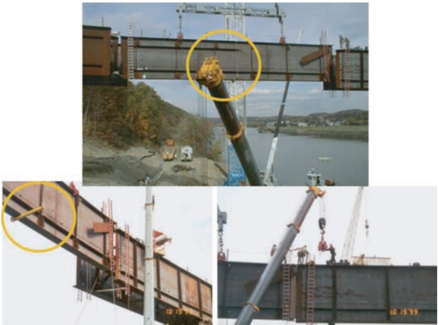
Figure 3-81. Ford City Bridge (EICCR11) installation of drop-in segment (Chavel, 2008).
