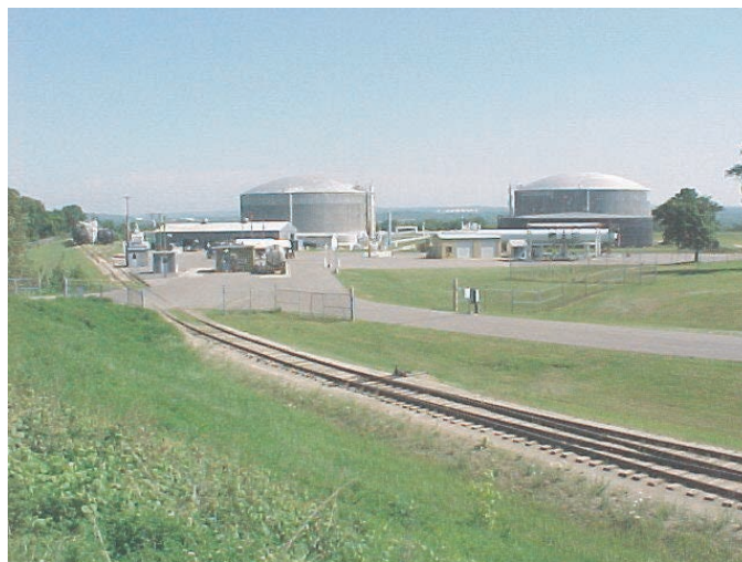
Figure 15. Example of an ammonia terminal (70).
