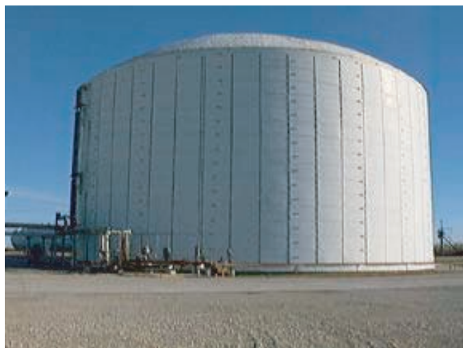
Figure 18. Ammonia storage tank (7).
