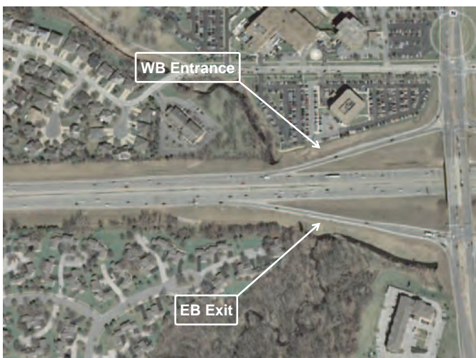
Figure 6. I-435/Quivira Rd—Ramps 1 and 12. (Image Credit: Google Earth™ Mapping Service).
