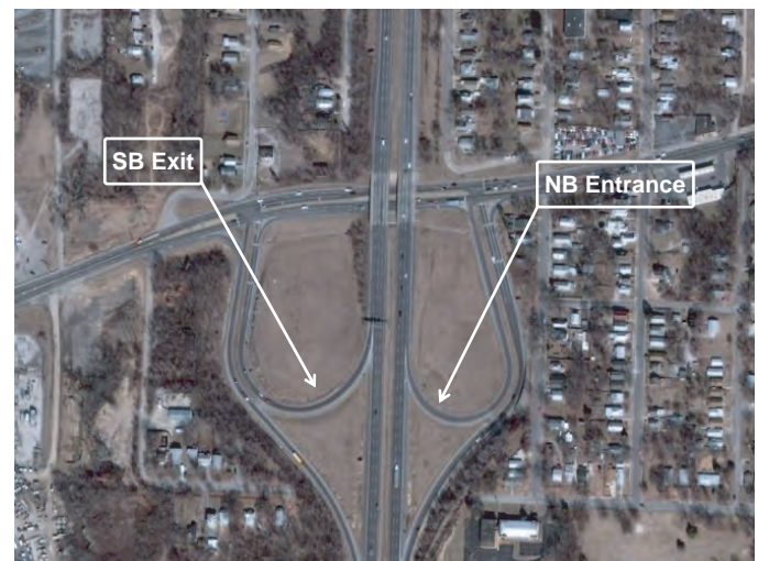
Figure 7. I-435/US 24—Ramps 2 and 15. (Image Credit: Google Earth™ Mapping Service).
