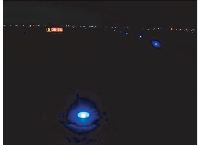
FIGURE 5 LED in-pavement taxiway edge light.
