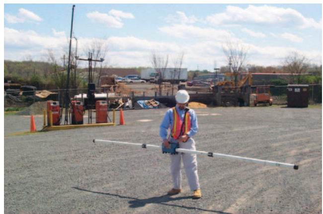
FIGURE 7 Terrain conductivity device. (Photo courtesy of So-Deep, Inc.)
