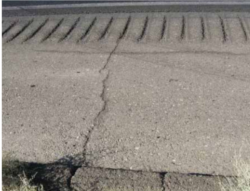
FIGURE 6 Prepavement condition of I-5 AR chip seal project.
