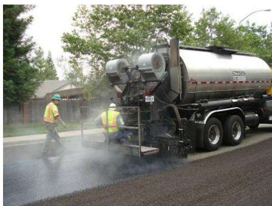
FIGURE 2 Spray application of AR binder at reduced temperature.
