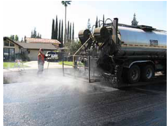
FIGURE 8 Application of AR binder with warm-mix engineering additive.
