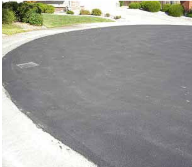
FIGURE 10 Cul-de-sac Scott Mills Court after slurry seal repair in October 2011.
