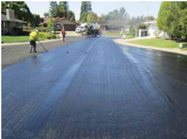
FIGURE 8 Application of AR binder with warm-mix engineering additive.
