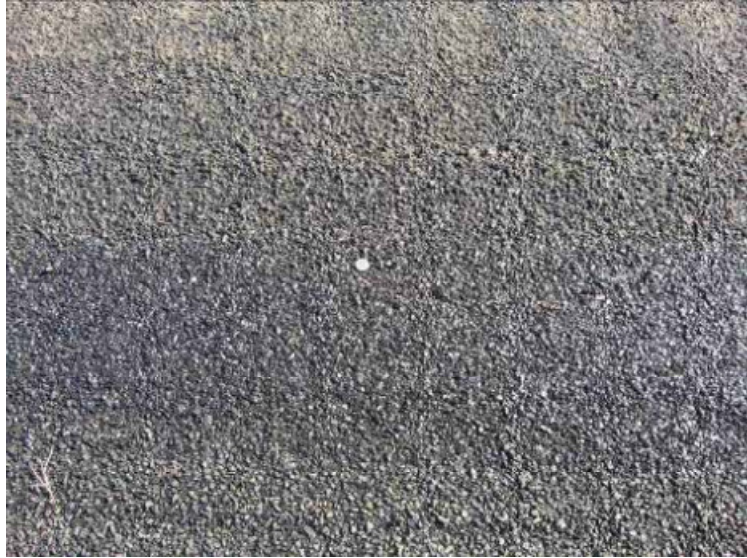
FIGURE 7 Completed AR with warm-mix chip seal project on I-5.
