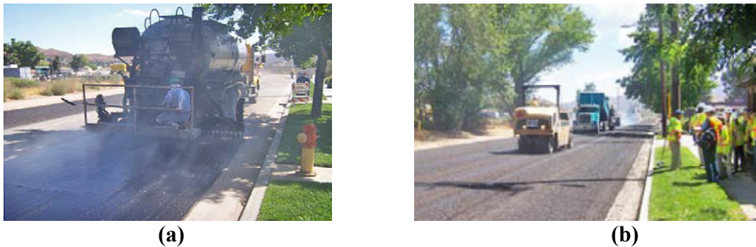
FIGURE 4 Spray of AR binder: (a) rock spreader and (b) compaction.
