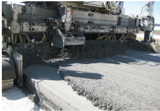
A thin, optimized surface lift is placed on a two-lift concrete pavement demonstration project on I-70 in Kansas.
