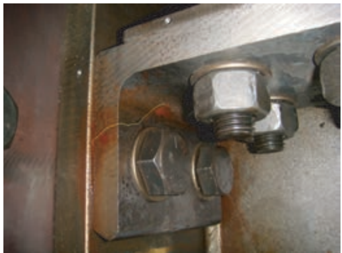
Figure 67. Typical fatigue cracks in single-angle retrofits (cracks marked with line).
