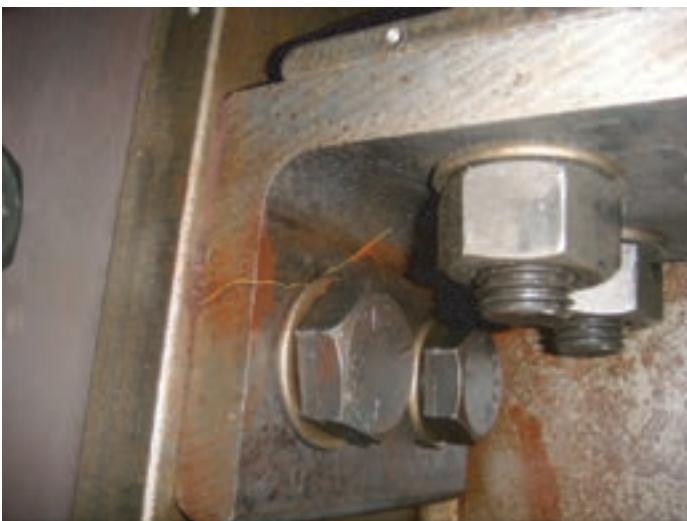
Figure 67. Typical fatigue cracks in single-angle retrofits (cracks marked with line).
