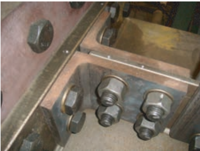
Figure 66. Typical double-angle and single-angle retrofits.
