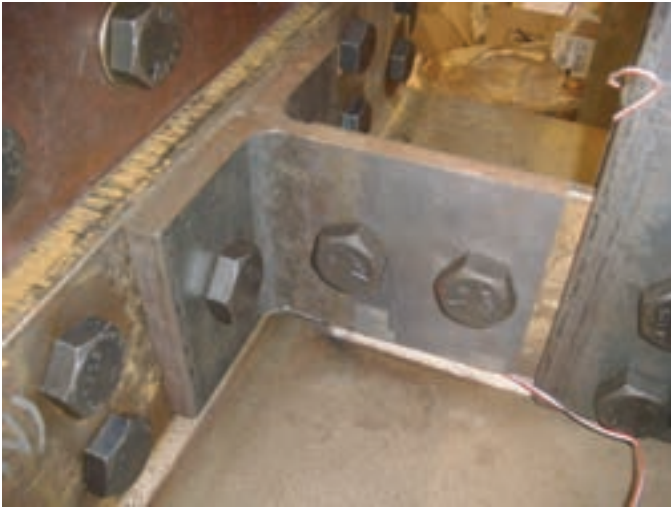
Figure 65. WT retrofit installed with reduced number of bolts.
