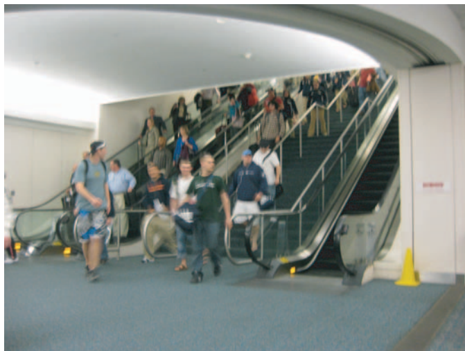
Figure 4-4. Escalator and stairs to baggage claim, MCO airport.
