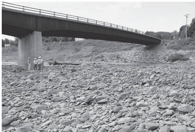
Figure 3.23. Schoharie Creek at State Route 161 about 4 miles upstream from I-90 Bridge. Boulder armor layer here is similar to the channel at I-90 before the bridge failed in 1987.
