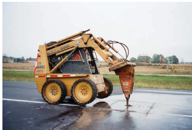
Trench excavated along the LTPP Wisconsin test section 55-0113. The HMA layer was supposed to be about 5-in. in thickness. It was found to be over 14-in. in thickness. The thinner test sections had the lower rut depths without the asphalt-treated base layer.
