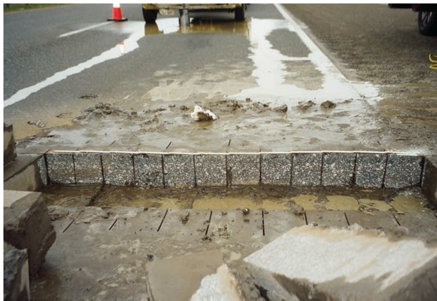
Left: Trench excavated within section 48-0507 (virgin mixture)
