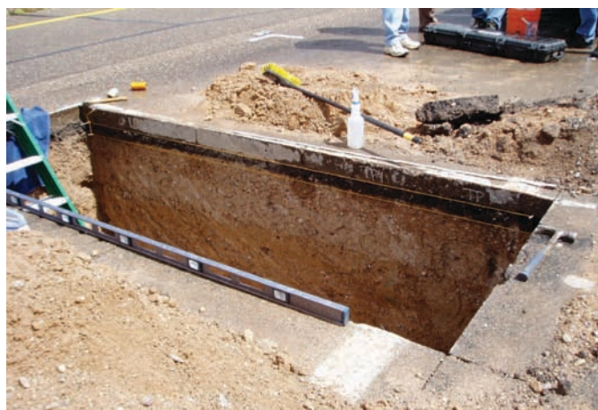
Figure 27. Forensic investigation of the Arizona SPS-5 project.
