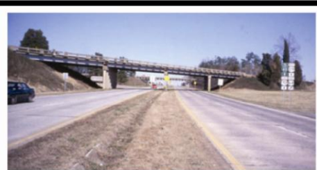
Figure 4.7. Historic Roads Need to Have Integrity As Well As Significance. I-85 Business at Lexington, North Carolina, built in the early 1950s, was one of that state's earliest limited-access freeways and was subsequently taken into the interstate highway system. An assessment of its integrity was critical to understanding the road as a historic structure and the refinements in roadway geometry that made it a "superhighway" in its time. The interchanges were considered so novel in this rural state that the department issued instructions to drivers about how to use exit and entrance ramps. This photo illustrates the median and shoulder treatments that were features of the original design. The roadway has significance within the statewide context of post-World War II urban bypasses. It remains largely as originally designed and meets the aspects of integrity. Photograph J.P. Harshbarger
