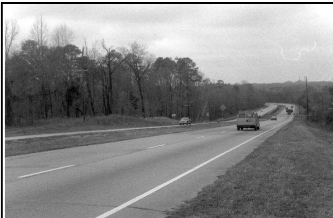
Figure 4.10. Historic Planned/Engineered Road US 27/Fort Benning Road (Georgia) Significance: First balanced-design road in Georgia applying federal-developed concepts, influenced all later designs and set standard that would be used over and over again on all later dualized (four-lane with median) highways (Criterion C). Significance established through statewide historic context for dualized highways. Integrity: Since balanced design is source of historical significance, location, design and association are the important aspects of integrity to consider. Significant features of road: design philosophy: design controls - speed, sight distance, grade, control of access all balanced in relationship to one another. Reflected in vertical and horizontal alignment, cross-sections, curve radii, use of a median, and construction of grade separation bridges located at points where military post roads could have access to the high-speed highway. Less significant features are the original pavement, shoulder treatments, side slopes, and railings.
