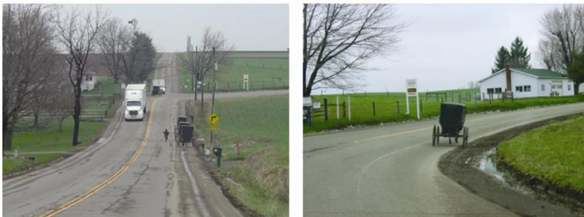
Figure 5.8. There is a wide range of flexibility for shoulders depending on local conditions. One of several treatments could be applied to increase the safety and operations of this segment of state highway for its multi-modal uses, including incremental widening of the travel lanes and shoulders, which in this locale also serve as a buggyway. Note that even the buggies off track on the inside of the curve. Enhanced pavement markings could improve the ability of motorized vehicles to stay in the appropriate travel ways, especially on the inside of the curve as buggies labor up the hill. Photographs M. McCahon.
