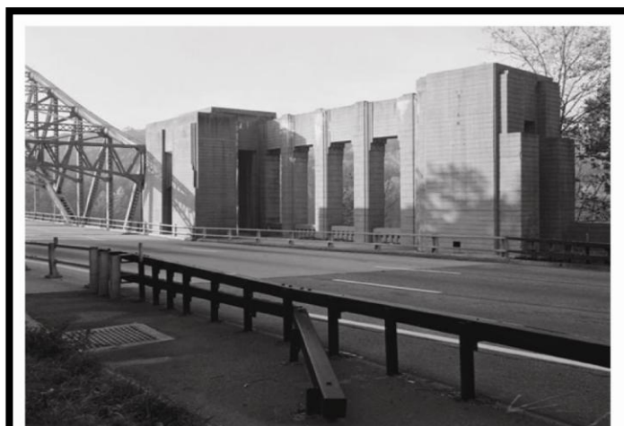
Figure 5.18. Barriers are an appropriate treatment to shield a historically significant object or fixture. Here barriers are placed between the roadway and the Art Deco-style pedestrian overlook at the Croton Reservoir Bridge on the Taconic State Parkway in New York.
