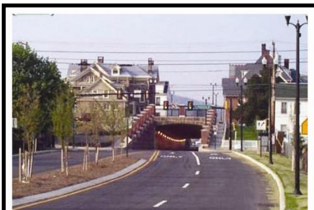
Figure 5.1. Depressed Roadway in Danville, PA Historic District. The depressed roadway takes the new river crossing approach road under, rather than through, the Danville, PA Historic District. Although the new road is a modern element introduced into the historic district, it represents an innovative, balanced solution that is scaled and detailed to be compatible while meeting the transportation need and purpose of the project.
