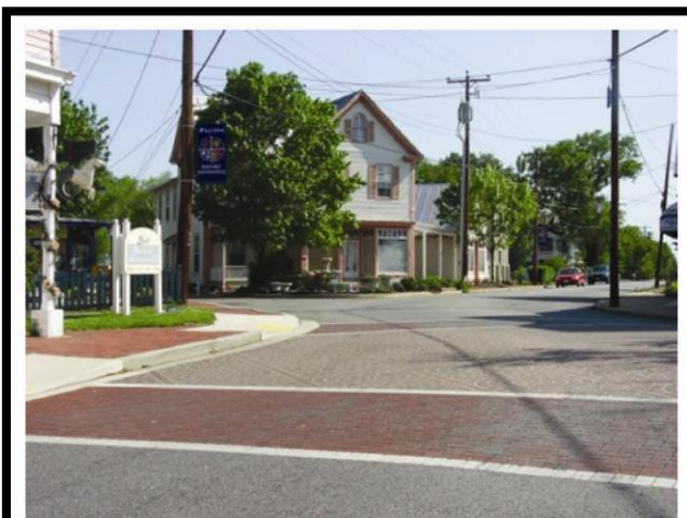
Figure 5.13. The stamped paisley pattern treatment and brick crosswalks added to a misaligned intersection with a vertical crest in the center of a small historic district is not only inappropriate from the historic perspective, it adds visual confusion to an already complicated intersection. Treatments that never existed in history should not be used in historic districts. It is more appropriate to use traditional pavement striping and signs. Photograph M. McCahon.
