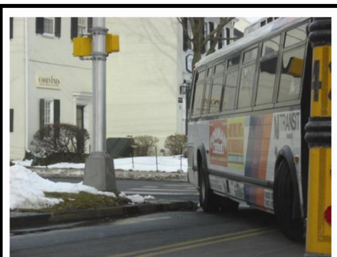
Figure 5.16. The design of intersections is significantly influenced by site-specific features or constraints as well as the potential users, from pedestrians to school and city buses. Shown here is a typical 90-degree street urban intersection within a historic district. Turning lanes and setbacks for traffic stopping lines have been installed, but the tracking of large vehicles still presents challenges. The basis for most of the geometric features is accommodating turning paths of the design vehicle to prevent off-tracking. Selection of the design vehicle is among the most important intersection-related considerations when working with historic roads. Photograph M. McCahon.
