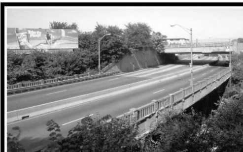
Figure 4.4. In response to the need to accommodate traffic approaching the 1923 Holland Tunnel through an already congested part of Jersey City, the New Jersey State Highway Department applied the economic theories of railroad location to a vehicular highway and built America's, and potentially the world's, first superhighway known historically as the Route One Extension. It is the quintessential engineered highway as it segregated through from local traffic and made provisions for changing grades along the limited-access, dualized highway that also passes through the Bergen Ridge as it approaches the at-grade tunnel portal. Most of its geometric features contribute to its historic significance. Because the highway was literally wedged into the existing fabric of Jersey City, the portion of the road from the tunnel to the south end of the Pulaski Skyway could not be widened. A completely new road on a new alignment (Jersey City Extension to the New Jersey Turnpike) was constructed in the 1950s to increase capacity. Its construction largely ensured that the historic road would retain its integrity. Photographer: Thomas Flagg.
