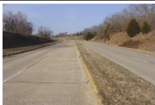
Figure 5.11. A concrete apron set into the integral curb on the concrete roadway is a historic treatment that appears to continue to function well given the condition of the bypassed section of US 66 in Missouri. Modern curbs and drop inlets would change the historic significance of the geometric design of the 1943 dualized highway. Photographs M. McCahon.
