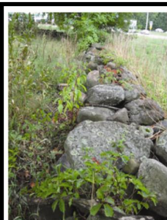
Figure 3.3. The dry laid rubble stone wall located near Chichester, NH was reconstructed in 1993 in accordance with the state DOT's administrative policy on rebuilding stone walls parallel to roadways. Photograph courtesy of Marc Laurin, NHDOT.
