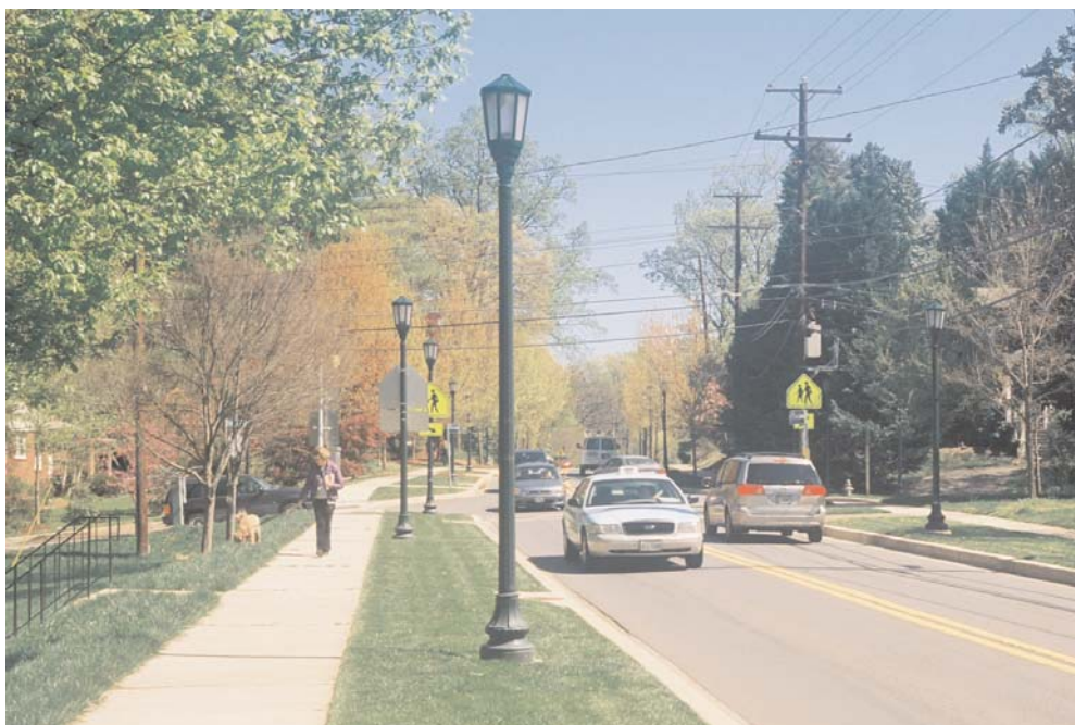
Improvement of MD 547, providing ADA-compliant sidewalks on both sides instead of a degraded walk on one side, was associated with nearly a 70 percent total pedestrian count increase
