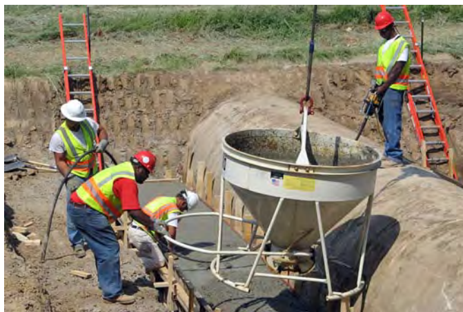
Figure 4-42. Red hats were worn by new job trainees for safety reasons to help all workers recognize them.
