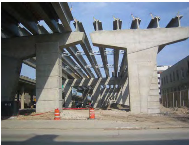
Figure 3-48. WisDOT increased levels of DBE participation through unbundling construction contracts.
