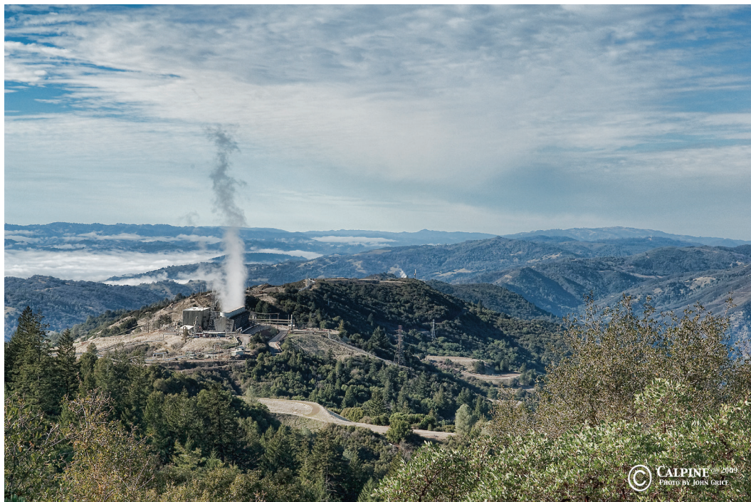
FIGURE 3.2 Ridgeline Unit 7 and 8 Power Plant (rated at 69 MW) in the left foreground at The Geysers in California. The turbine building, housing the two turbine-generator sets, the operator's control room, and various plant auxiliaries are on the left. The evaporative cooling tower with steam emanating from the top is on the right of the main complex. The beige pipelines along the roads (with square expansion loops) are the steam pipelines that gather the steam from the production pads and bring it to the plant. A high-voltage transmission line (denoted by lattice towers) is in the middle foreground of the picture. SOURCE: Calpine.
