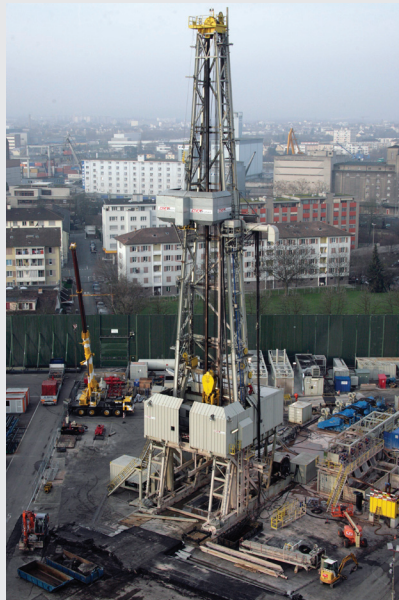
Figure 1 Drilling activity in the middle of the city of Basel. SOURCE: KEYSTONE/Georgios Kefalas.
