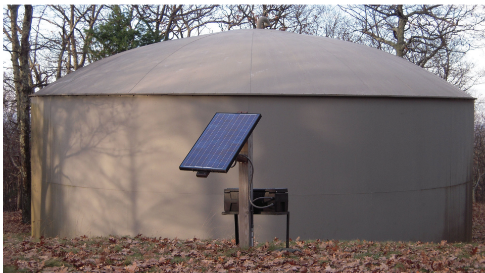
FIGURE 5.1 Small solar cell installation monitoring the water supply in Shenandoah National Park in Virginia.
