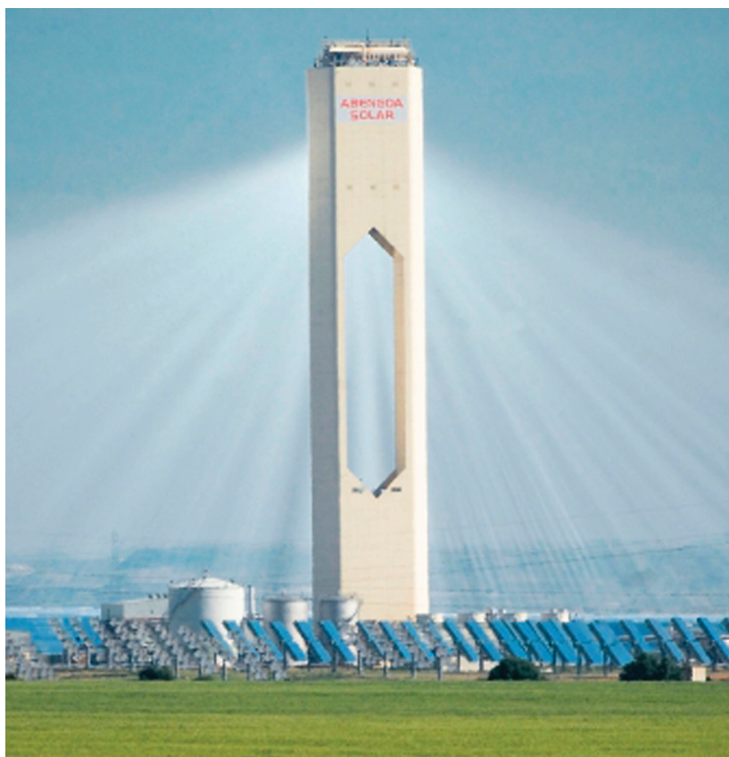
FIGURE 5.11 Eleven-megawatt Solar Power Tower near Seville, Spain. SOURCE: Courtesy of Abengoa Solar.
