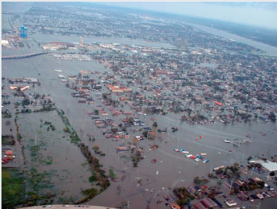
FIGURE 2-1 Aerial photograph of flooding as a result of breached levees in New Orleans in the wake of Hurricane Katrina.
