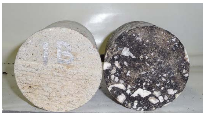
Figure 1.32. Core 1 from Station 0+35 in Section 1.
