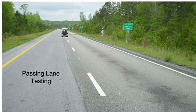
Figure 5.1. NPTT blind test location.
