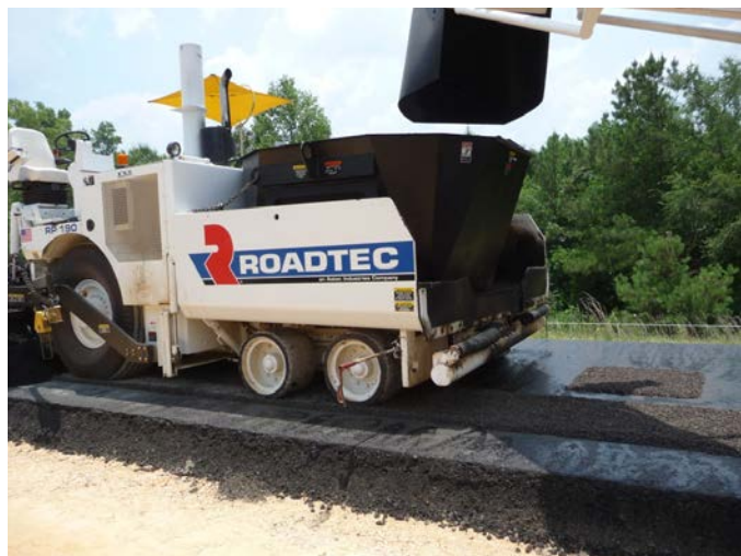
Figure 1.30. Paver moving into delaminated areas and using RAP materials in Section 6.
