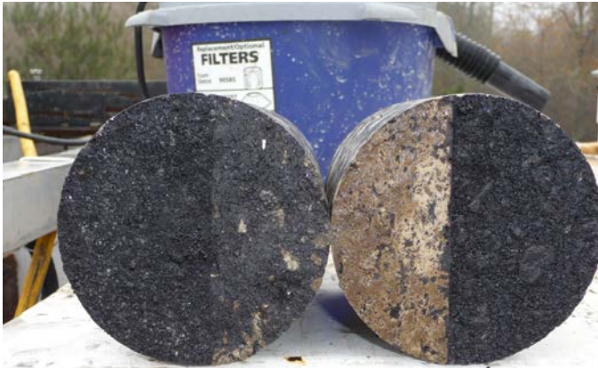
Figure 1.36. Core 5 from Station 2+20 in Section 9.
