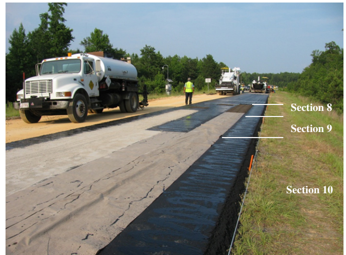
Figure 1.25. Brown paper and baghouse fines used at depth of 5 in. in Sections 9 and 10, near Section 8 (Figure 1.24 above).
