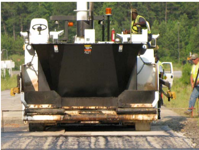
Figure 1.23. Brown paper (left) and baghouse fines (right) used as bond breakers in Section 1 at depth of 5 in.
