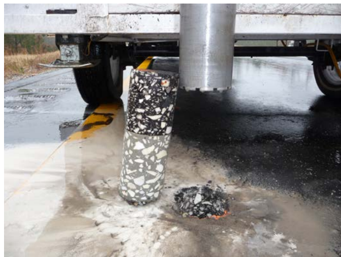
Figure 1.33. Core 2 from Station 0+45 in Section 2.
