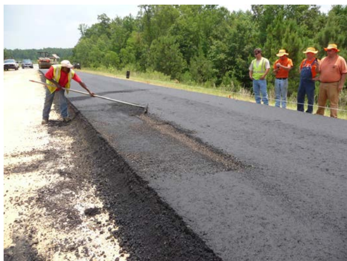
Figure 1.31. Paver pushing RAP materials to the surface in Section 6.
