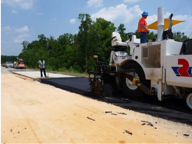
Figure 1.22. Concrete slab (Stations 0+15 to 0+65) and leveling HMA (Stations 0+65 to 2+65).
