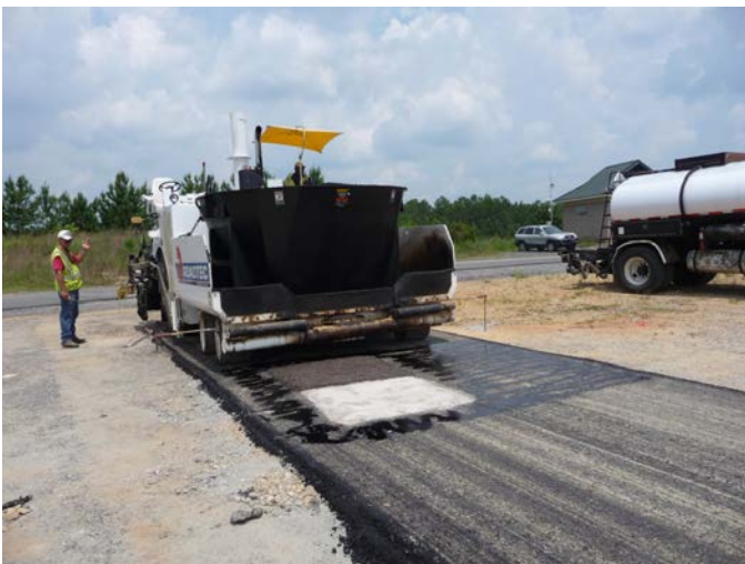
Figure 1.3. Two squares covered with baghouse fines and RAP materials.
