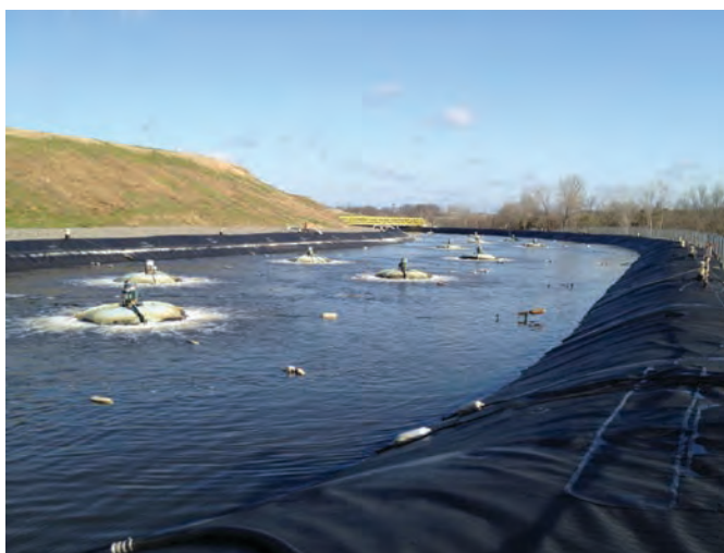
Figure 2. BNA treatment system.
