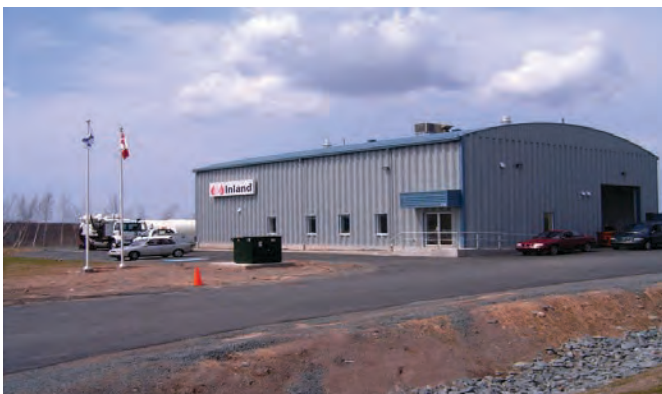
Figure 1. YHZ glycol recycling facility.
