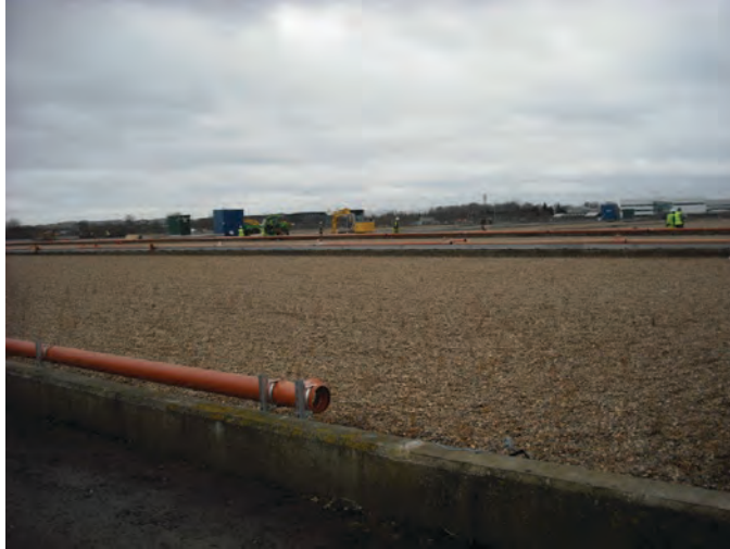
Figure 2. Retrofit of aerated gravel beds (reed beds).
