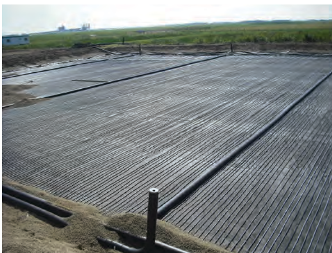
Figure 3. Installation of drain and aeration lines.
