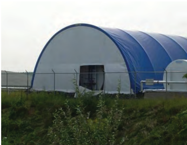
Figure 2. Low-concentration processing building.
