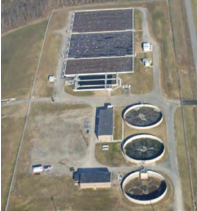
Figure 2. Aerial photo of CVG activated sludge treatment system (Photo courtesy of KCAB).
