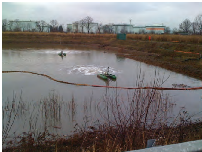
Figure 3. Aeration in main reservoir.
