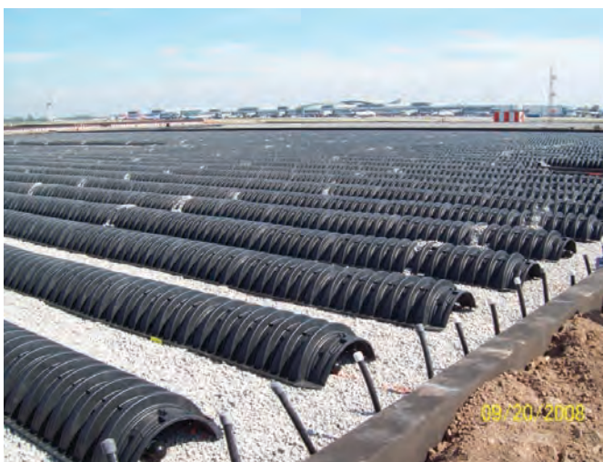
Figure 2. Construction of the BUF aerated gravel bed.
