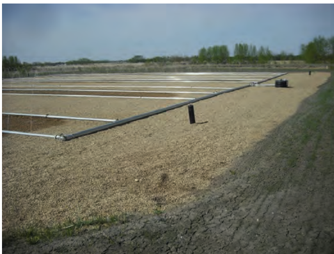
Figure 2. Vertical flow distribution system.
